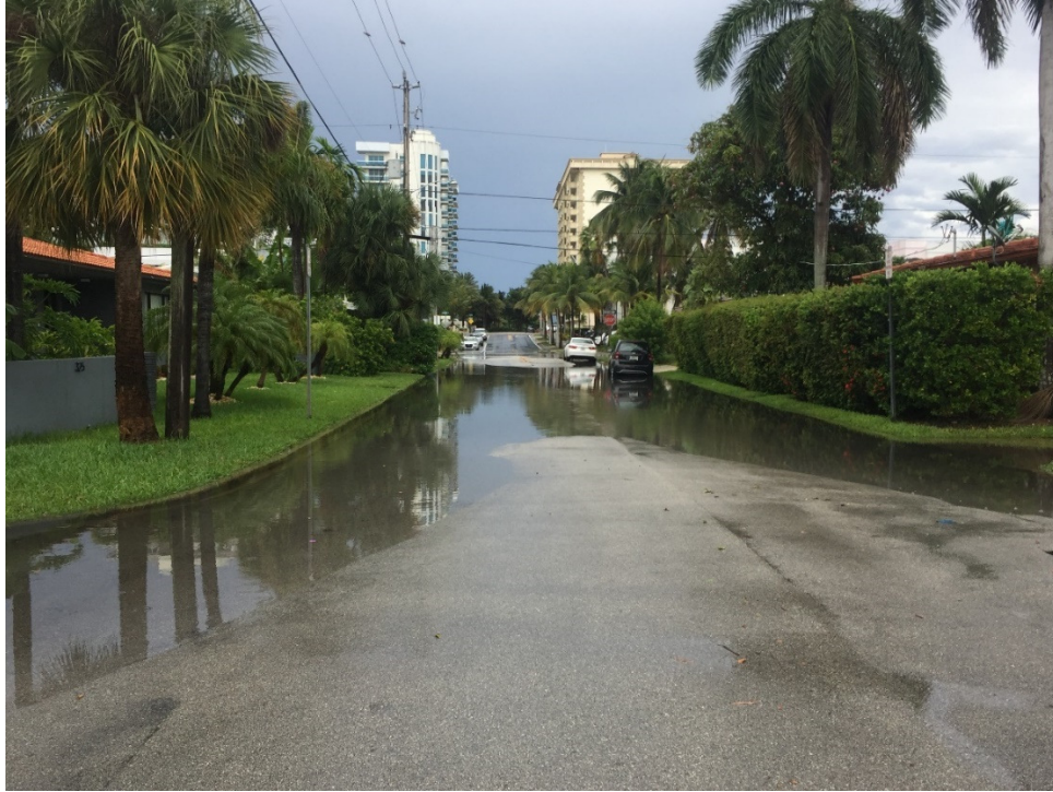
92 ND STREET AT ABBOTT AVE INTERSECTION, JULY 24, 2016 (ESTIMATED 1.50 INCHES OF RAIN PER SFWMD RAINFALL DATA)
