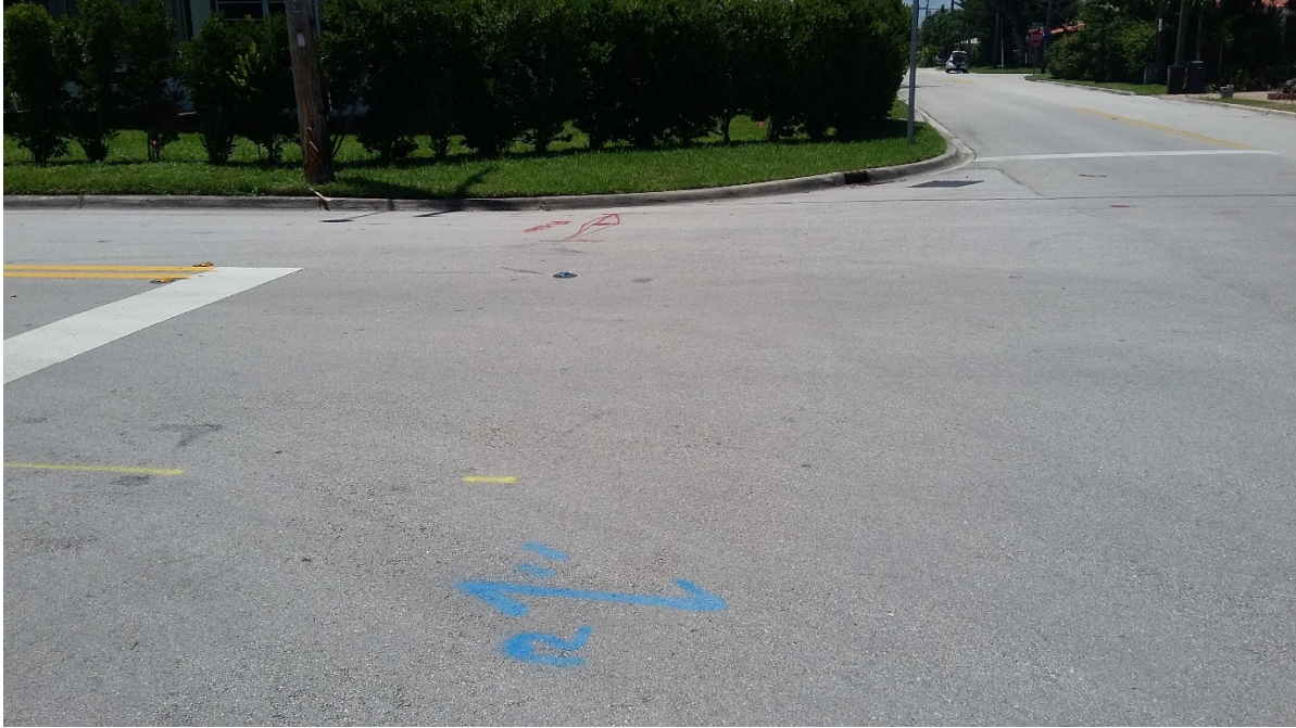
EXISTING GAS MAIN, WATER MAIN, FPL AND AT&T DUCT BANKS ALONG ABBOTT AVE
