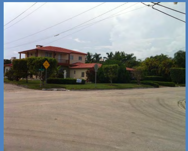
94 th Street at Bay Drive Existing Conditions
