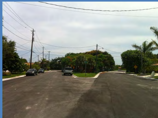
Bay Drive at Hawthorne Avenue Existing Conditions
