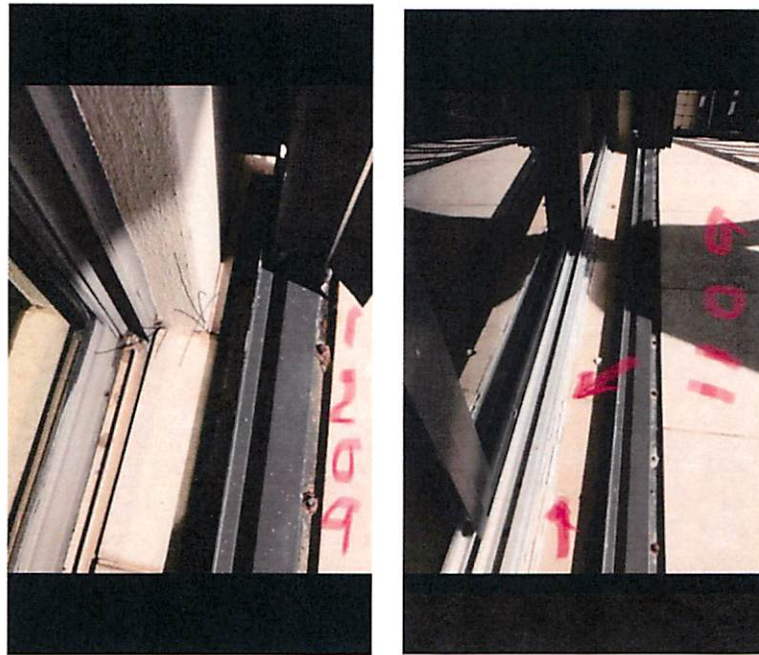
Figure A1: Exterior sealant past its serviceable lifespan at sealant between the window/door frames and masonry/concrete walls & balcony floors
