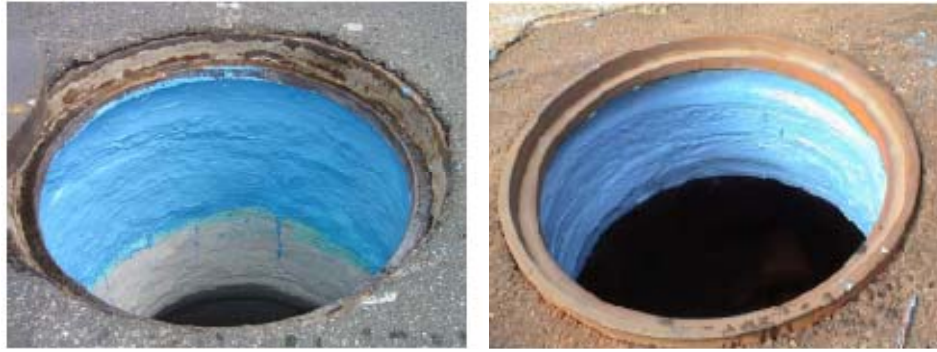
Figure 4.11 Chimney Seal Installed (Courtesy, USSI, Inc)
