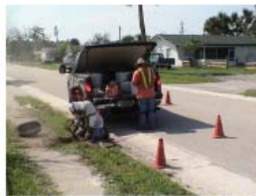
Manhole Frame / Chimney Sand-Blasted
