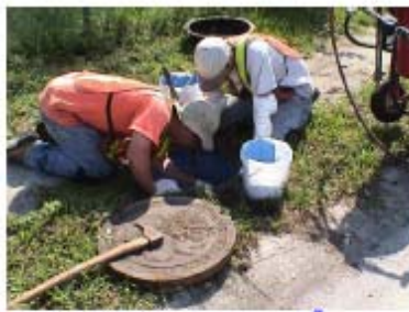
Frame & Chimney – Elastaseal® Coat
