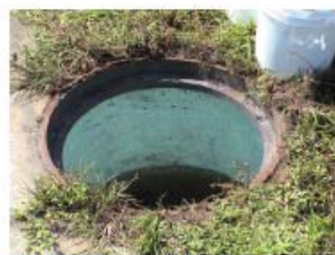
Frame & Chimney – Prime Coat
