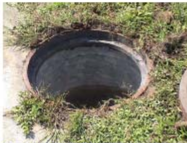
Manhole Interior Following Sand-blasting
