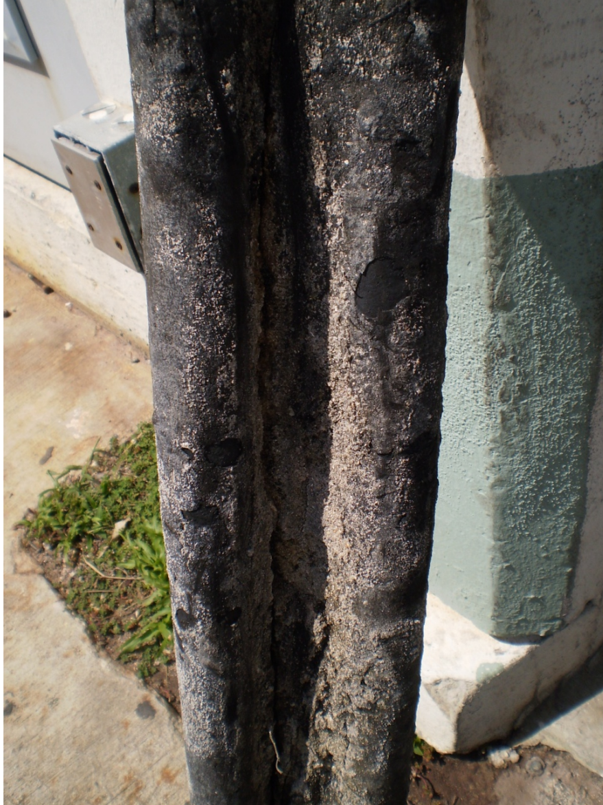
Figure 4.6 Example of Old Orangebrook Pipe in Very Deteriorated Condition
