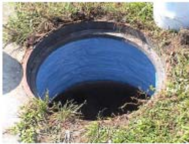
Manhole Following Abatement
