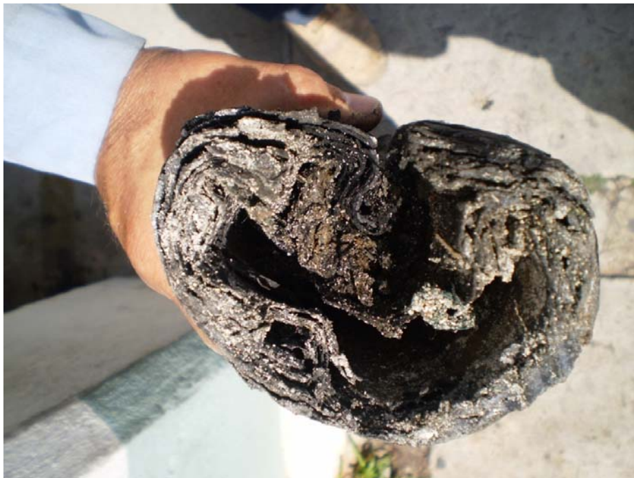
Figure 4.5 Example of old Orangebrook Pipe in Very Deteriorated Condition
