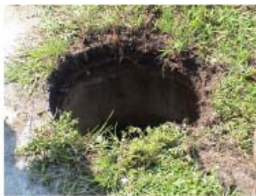
Manhole Prior to Abatement
