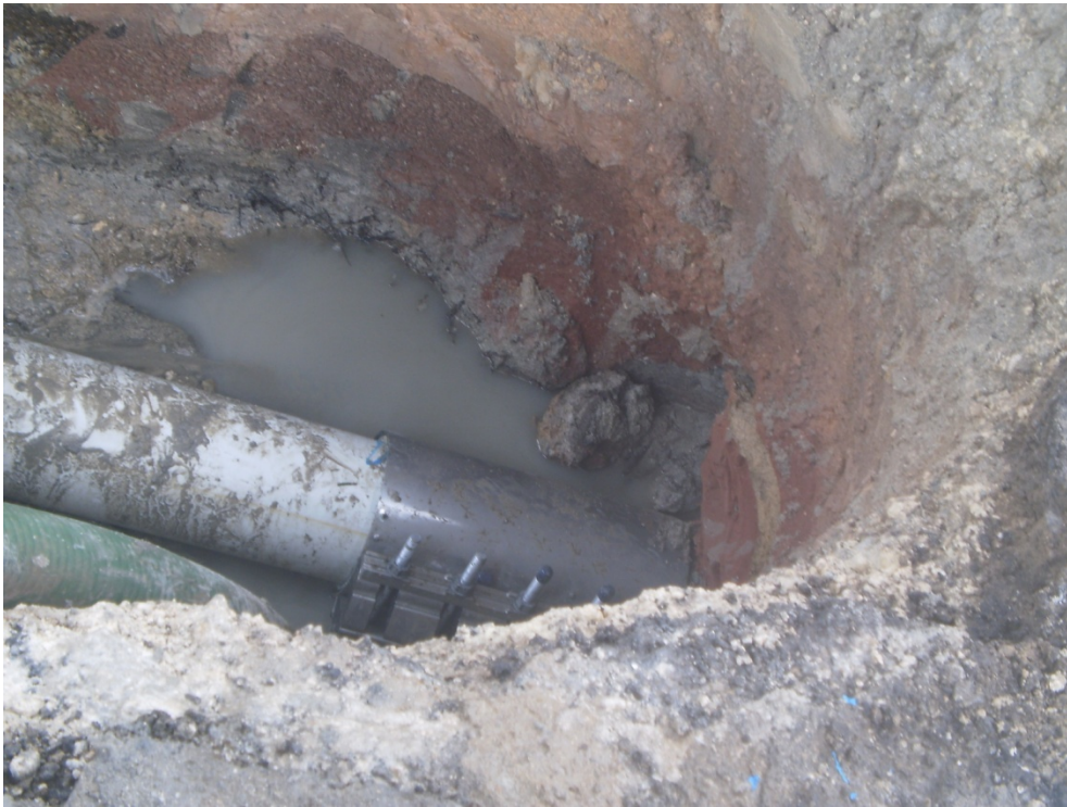
Figure 4.8 Example of old PVC Service Line – Many are in Deteriorated Condition and/or Broken
