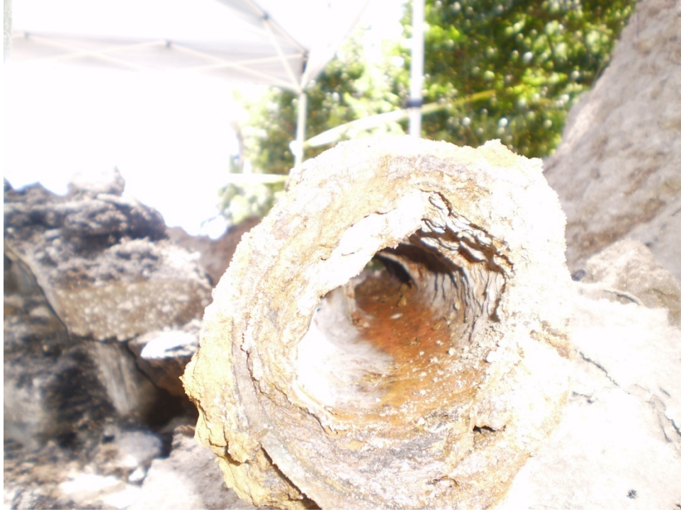
Figure 4.7 Example of Old Cast Iron Service Line in Very Deteriorated Condition – Exposed to Salt Water
