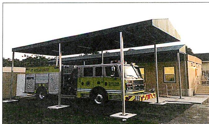
Temporary MDFR Palmetto Bay Fire Station #62
