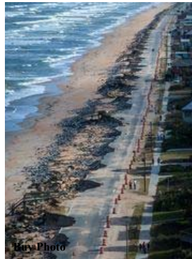
A section of State Road A1A in Flagler County shows erosion damage after Hurricane Matthew passed the east coast of Florida in October 2016. The section of road had been previously undermined, and county officials recently had begun a beach replenishment process. (Photo: David Albers/Naples Daily News)
