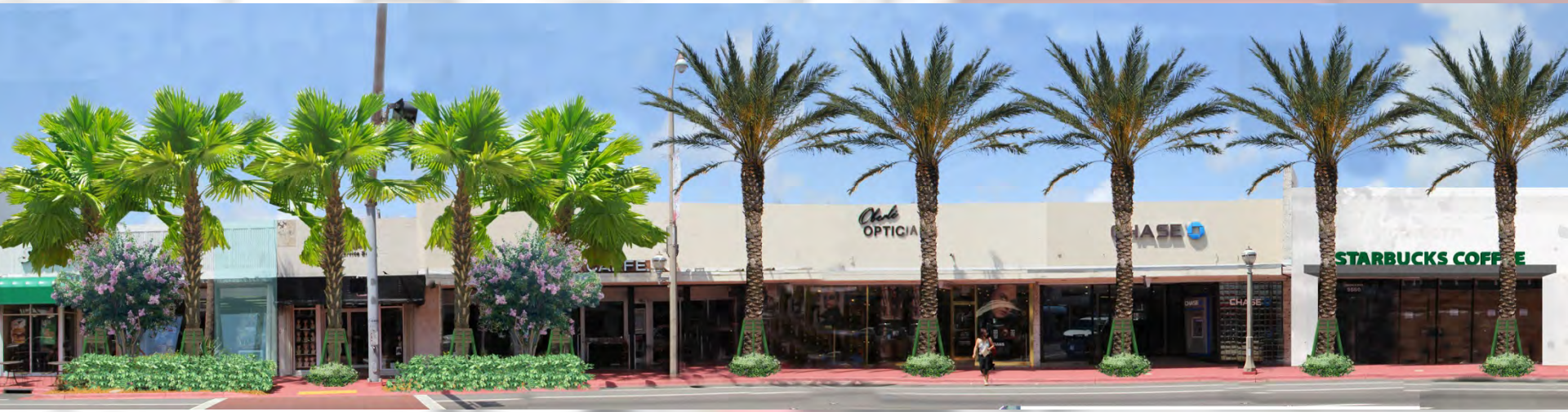
Harding Avenue – Proposed Date Palms With Temporary Bracing Original Scope of Work
