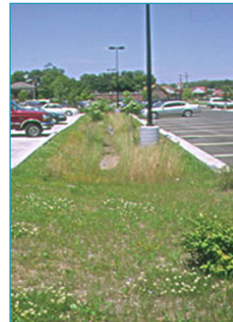
The Discovery Center parking lot features bioswales planted with native species that filter pollutants from parking lot runoff.
