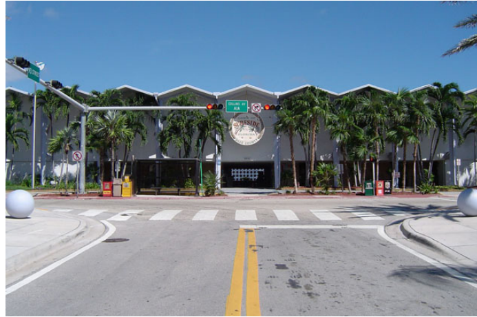
1. EXISTING COMMUNITY CENTER The current center masks the greatest asset of the Town of Surfside, the ocean.
