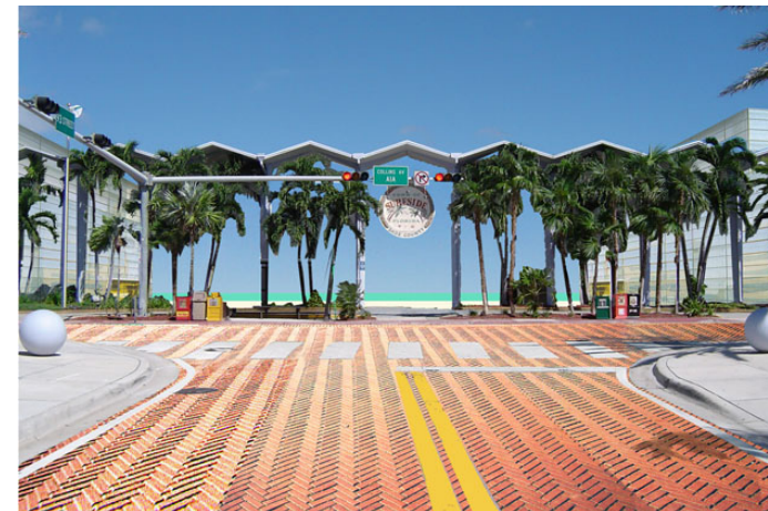
4. REASSIGNMENT OF FUNCTIONS Community Center function and administrative space could be reconfigured in a number of ways that would allow for views through to the beach and provide the community with an open and inviting place to spend time.
