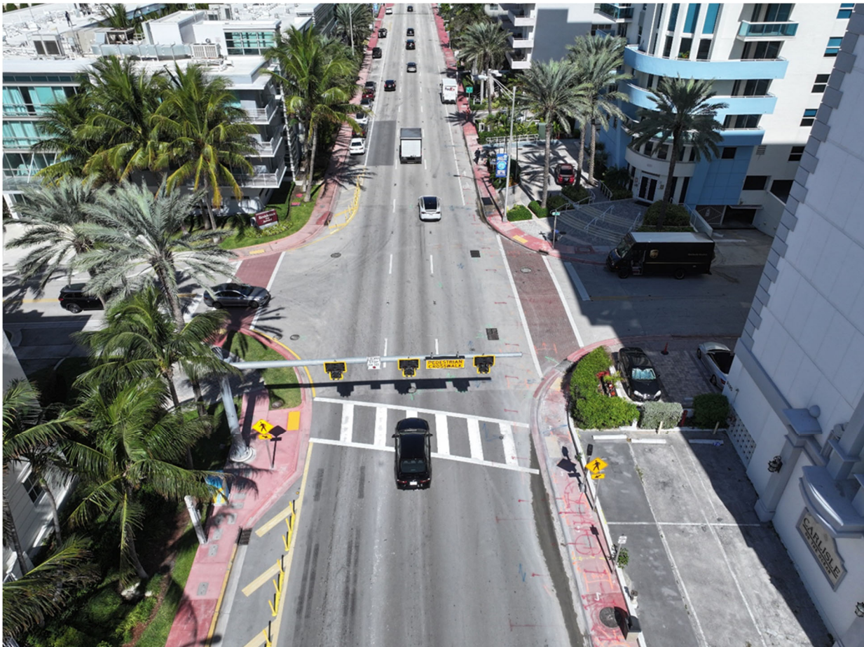
Figure 43 State Road A1A/Collins Avenue at 92 nd Street
