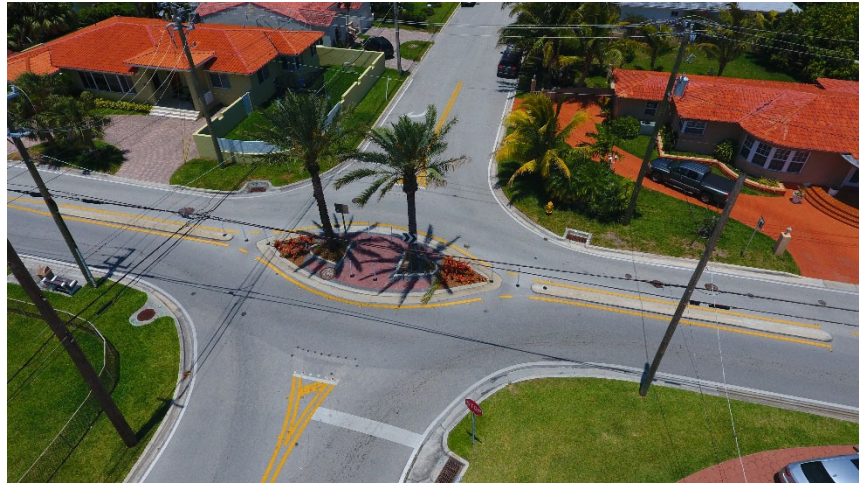
Figure 3 Intersection of Byron Avenue and 88 th Street
