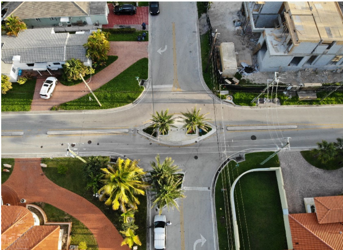
Figure 31 Median Diverter at the 88 th Street and Byron Avenue intersection
