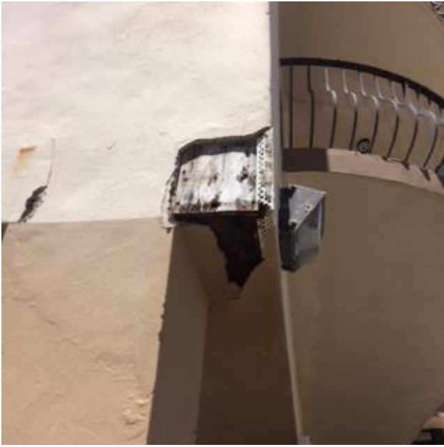
Figure 5: Delaminated stucco
