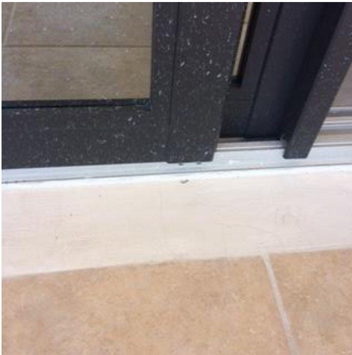
Figure 1: Cracking at balcony floor slab at sliding door threshold
