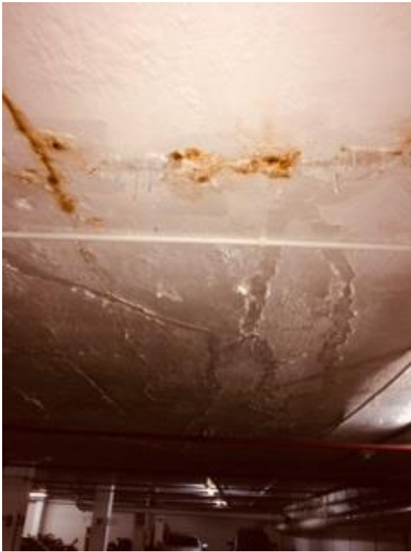
Figure 2: Hairline cracking at underside of floor slabs in garage
