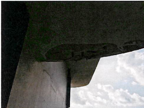
Figure C: Concrete spall at balcony slab edge in units 1008 & 211
