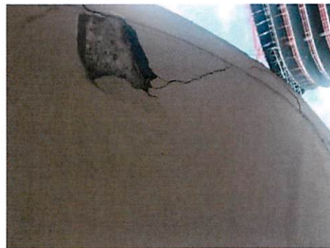
Figure C: Concrete spall at balcony slab edge in units 1008 & 211
