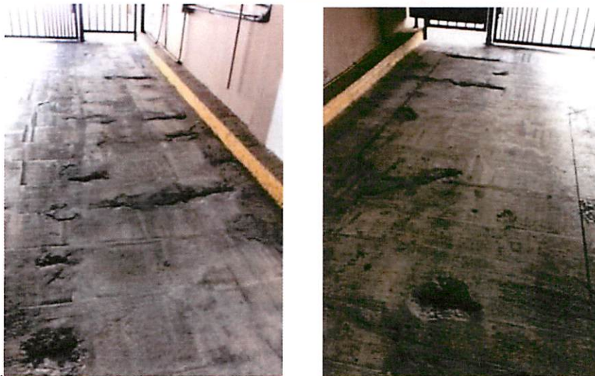
Figure J2: Spalling with exposed steel reinforcement at top of garage deck.
