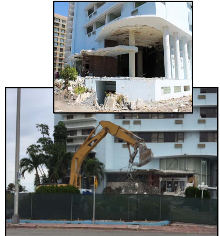
TERRA GROUP DEVELOPMENT – Eighty-Seven Park Demolition begins Jan 6 th , without fencing and protective green mesh. By Jan 12 th , they added the fence
