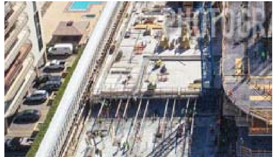
BELOW GRADE PARKING GARAGE
