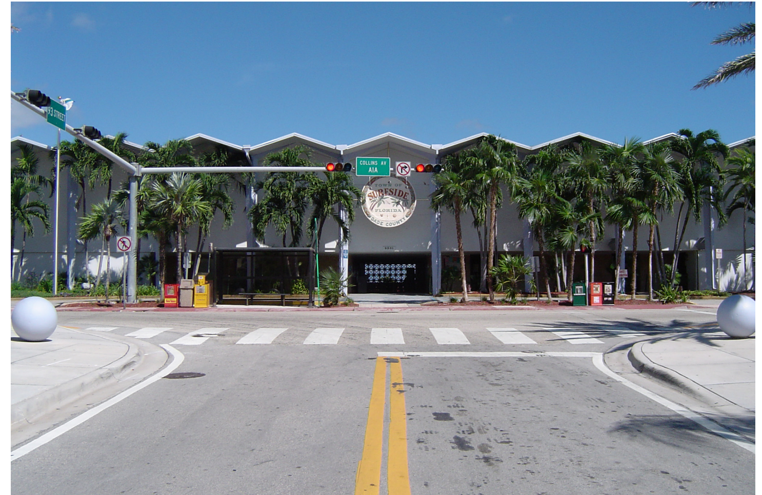
ABOVE: EXISTING COMMUNITY CENTER RIGHT: EXISTING TOWN HALL
