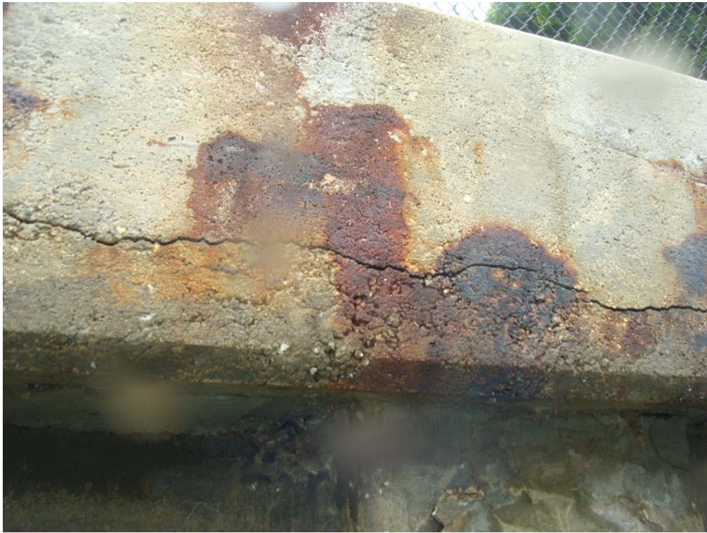
Photo 12.5: Longitudinal Spall Cracking in Cap, Rusted Reinforcement
