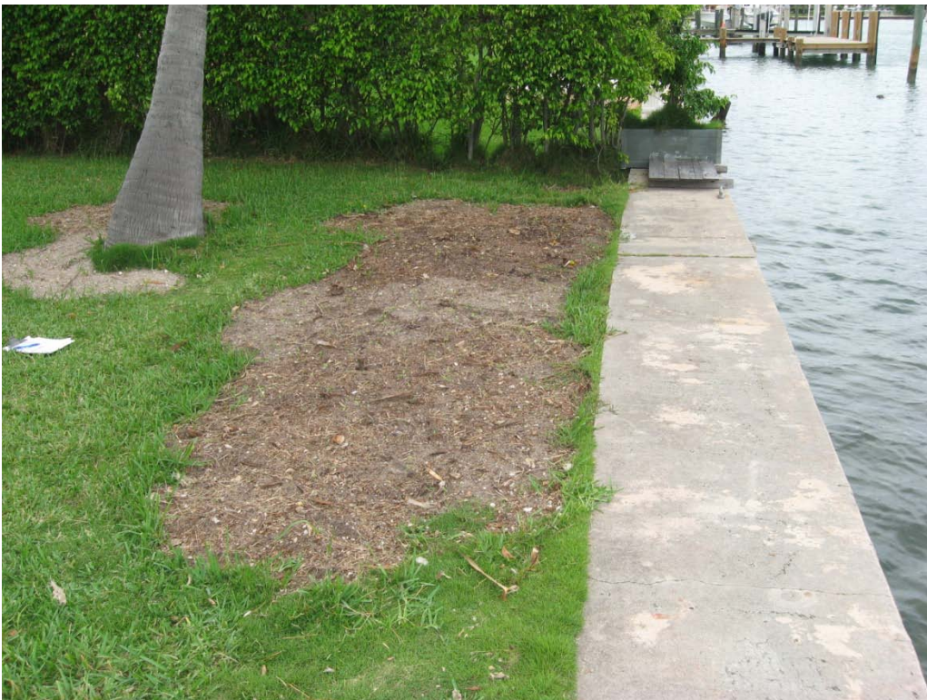
Photo 2.2: Recently Placed Imported Fill
