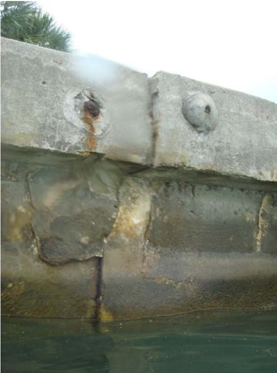
Photo 9.2: Vertical Shear Crack in Wall Face and Cap
