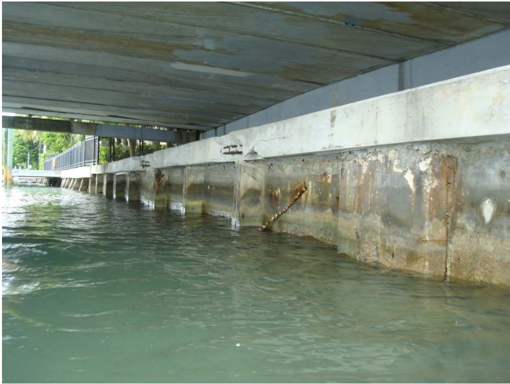
Photo 12.7: Longitudinal Spall Cracking in Cap beneath FDOT Bridge
