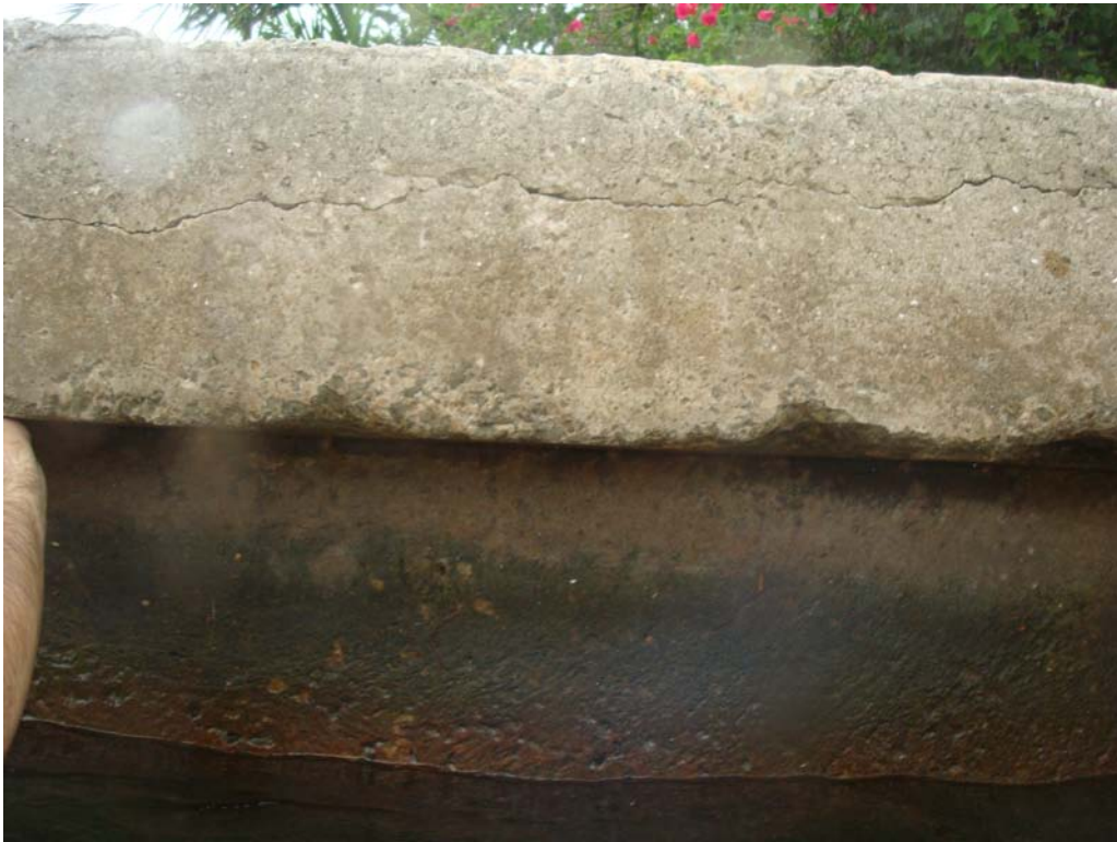
Photo 10.1: Longitudinal Cracking Along Cap
