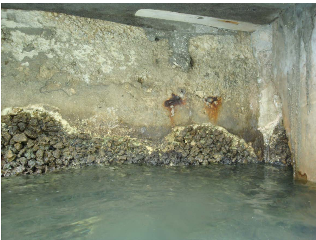
Photo 5.5: Degraded Concrete Sheet Piles
