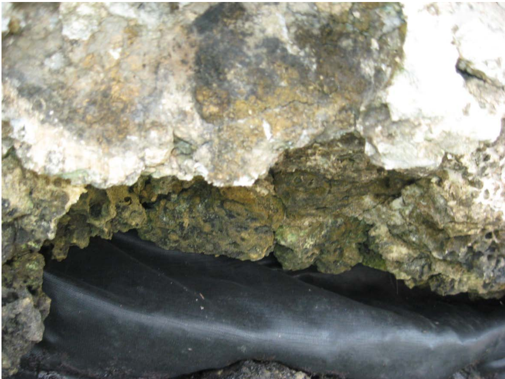
Photo 1.3: Geofabric Witnessed Through Wall
