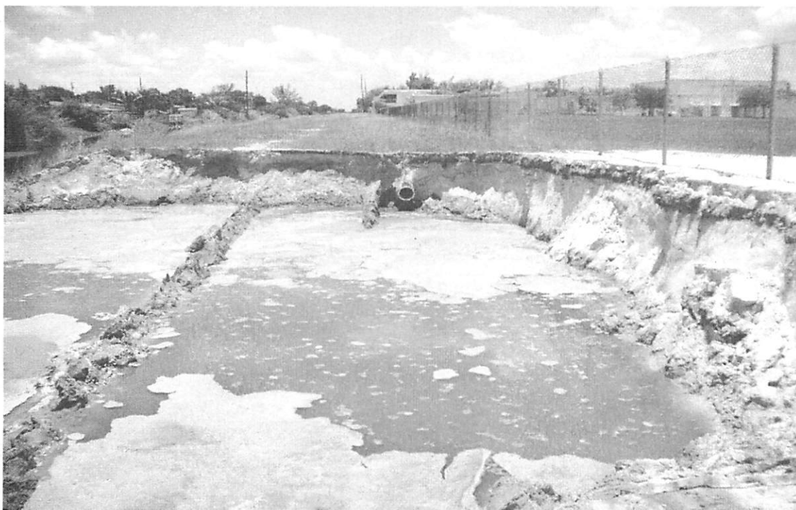
72-inch Pre-Stressed Concrete Cylinder Pipe Break at Biscayne Canal & NW 17 Avenue
