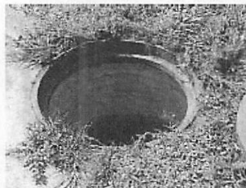
Manhole Interior Following Sand-blasting
