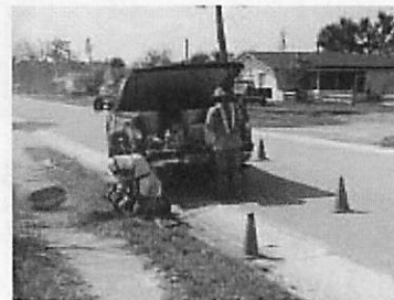
Manhole Frame / Chimney Sand-Blasted
