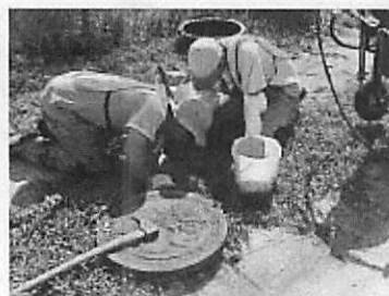
Frame & Chimney – Elastaseal® Coat
