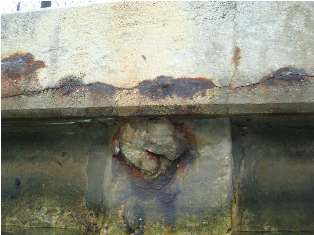
Photo 12.2: Longitudinal Spall Cracking in Cap, Rusted Reinforcement
