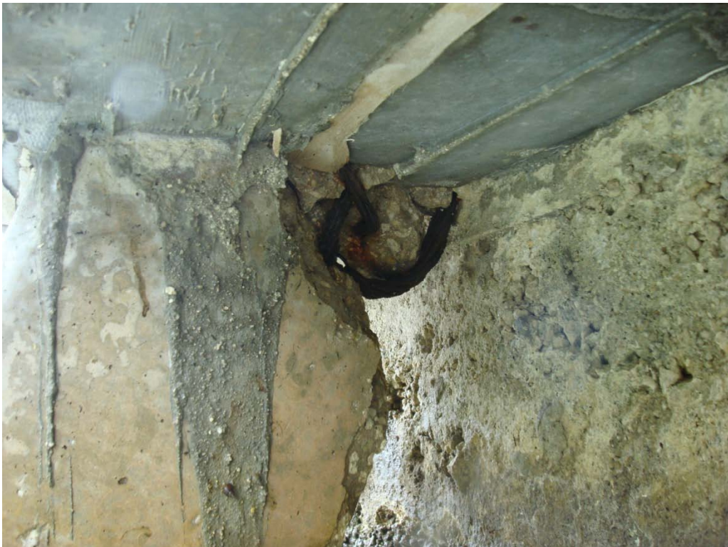
Photo 5.2: Exposed Steel Reinforcement in Batter Pile
