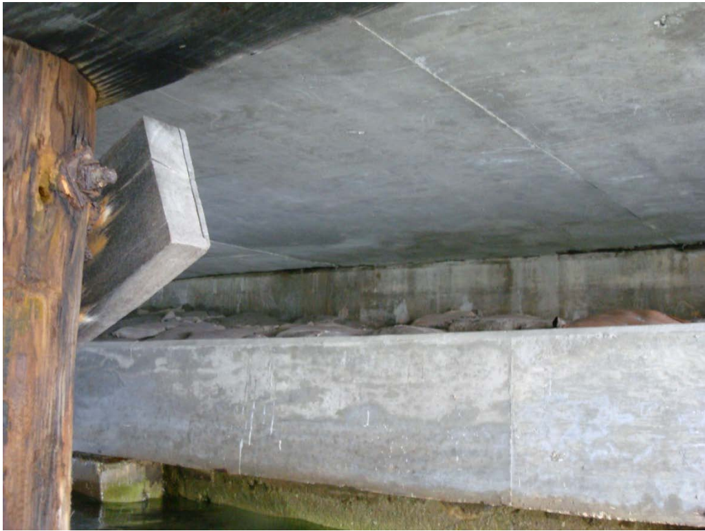
Photo 3.1: Concrete Cap In Front of Abutment with Backfill
