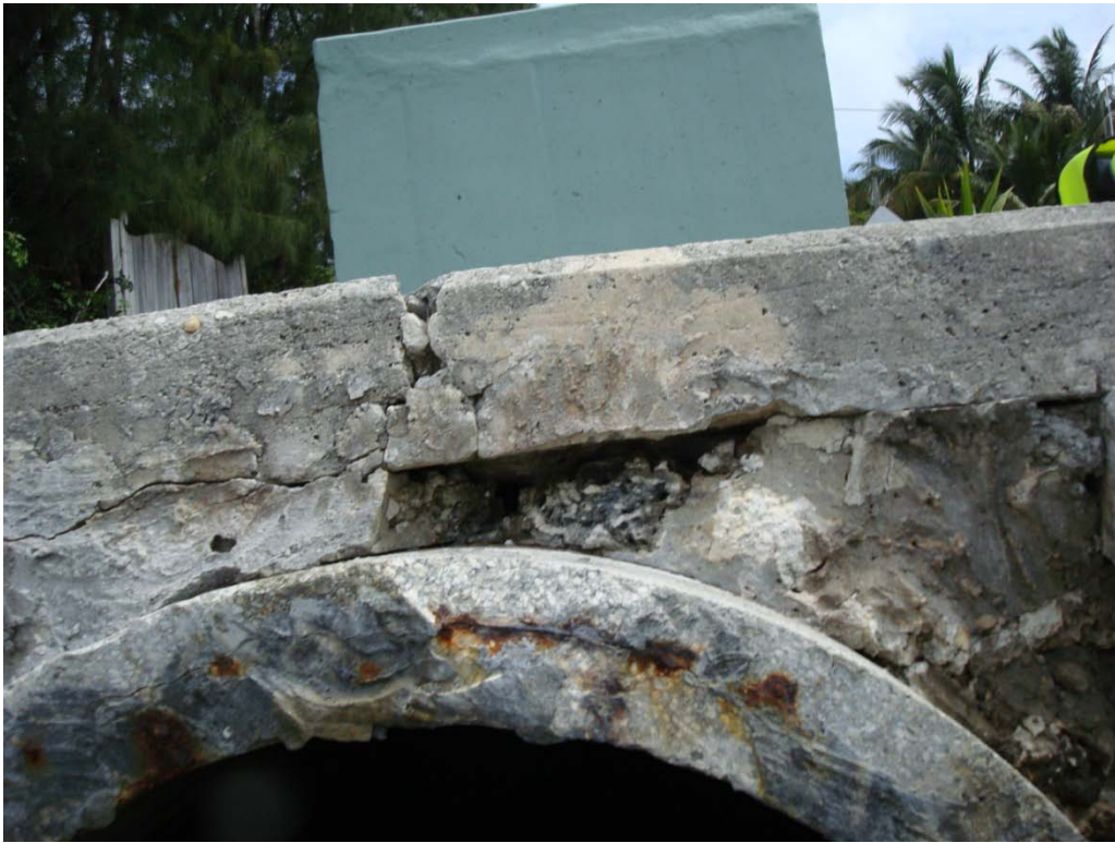
Photo 1.2: Crack above Concrete Outfall
