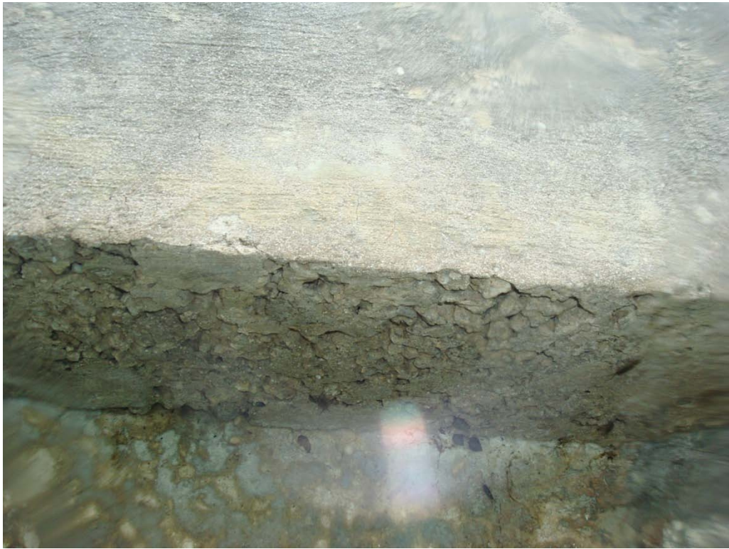
Photo 9.1: Honeycombing in Concrete Cap
