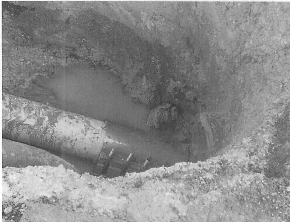
Figure 4.8 Example of old PVC Service Line – Many are in Deteriorated Condition and/or Broken
