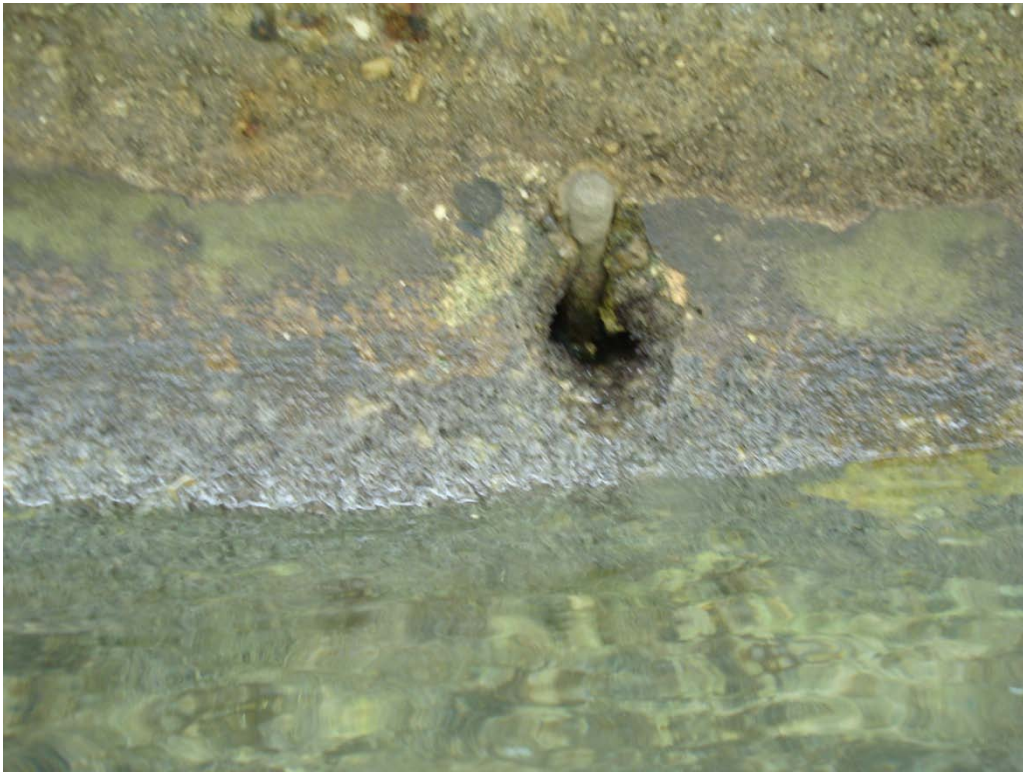
Photo 5.1: Tie Rod Pulled Through Sheet Pile
