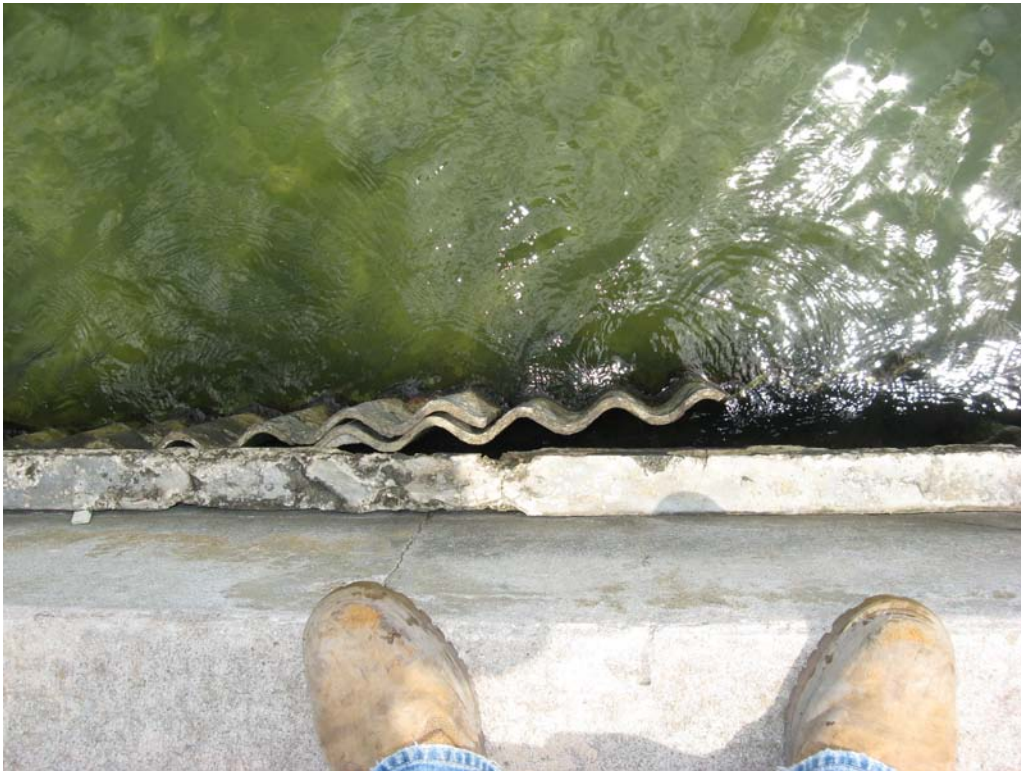
Photo 2.2: Asbestos-Concrete Sheet Piles In Front of Wall
