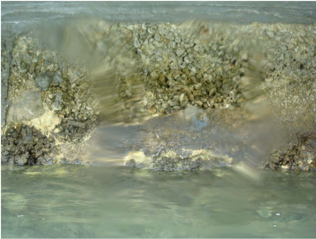
Photo 5.3: Degraded Concrete Sheet Piles
