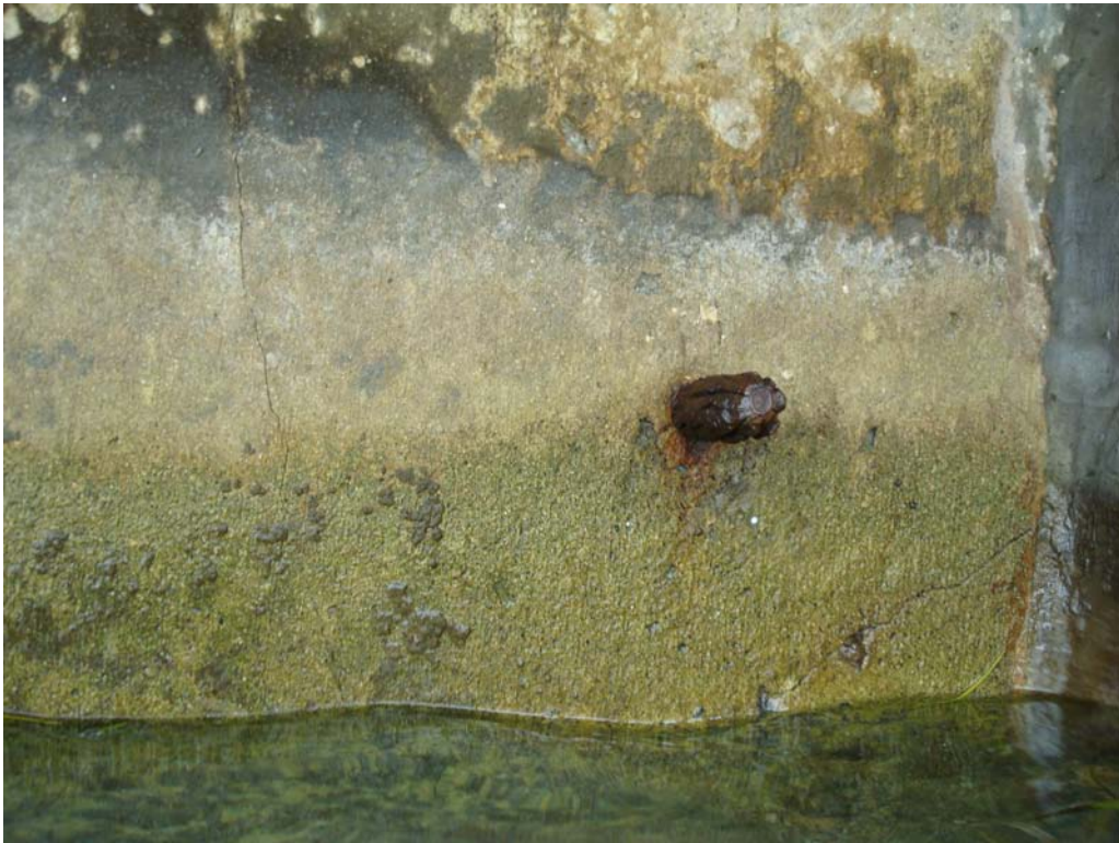
Photo 8.1: Rusted Tie-back Rod End
