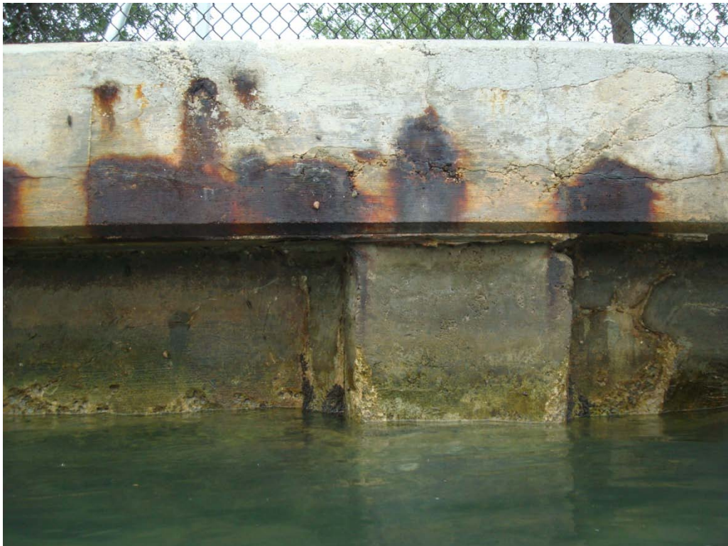
Photo 12.6: Longitudinal Spall Cracking in Cap, Rusted Reinforcement
