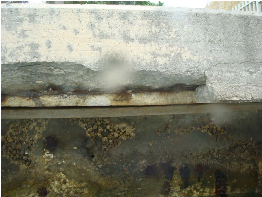
Photo 11.3: Degraded Sheet Piles, Spalling Cap
