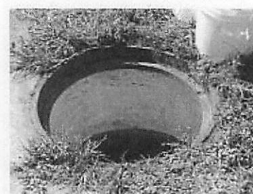
Frame & Chimney – Prime Coat
