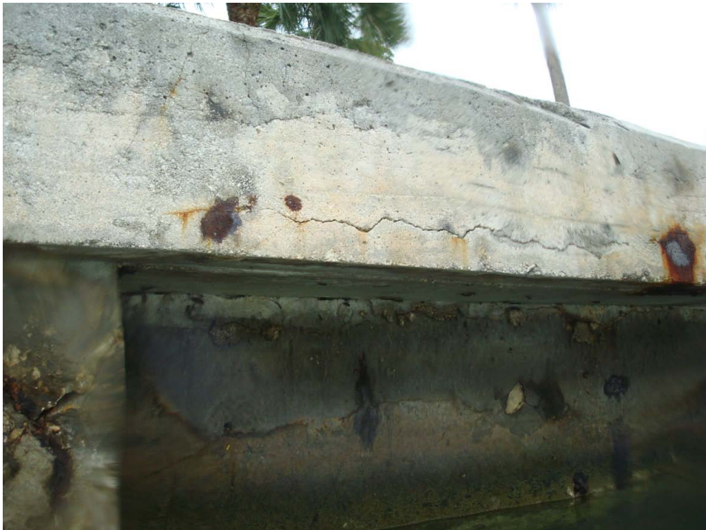
Photo 11.6: Spall Cracking in Cap, Rusted Reinforcement
