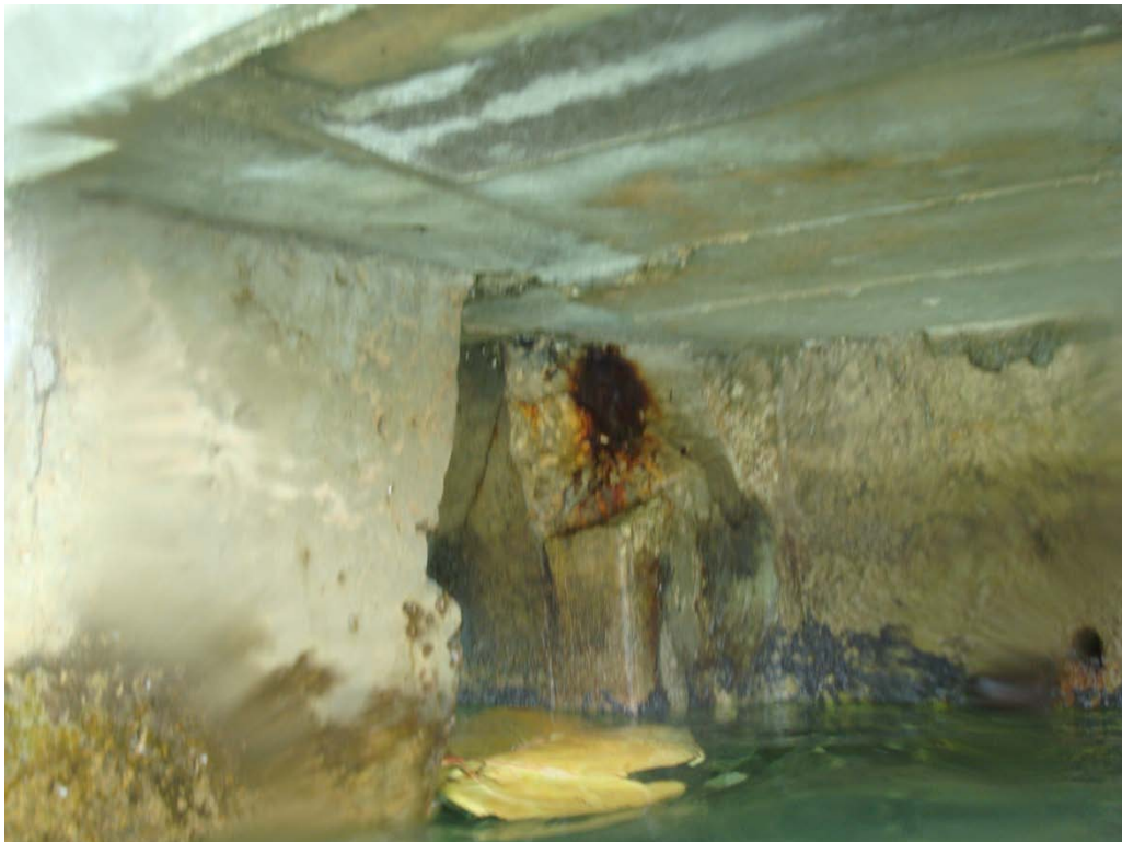
Photo 6.2: Exposed Steel Reinforcement
