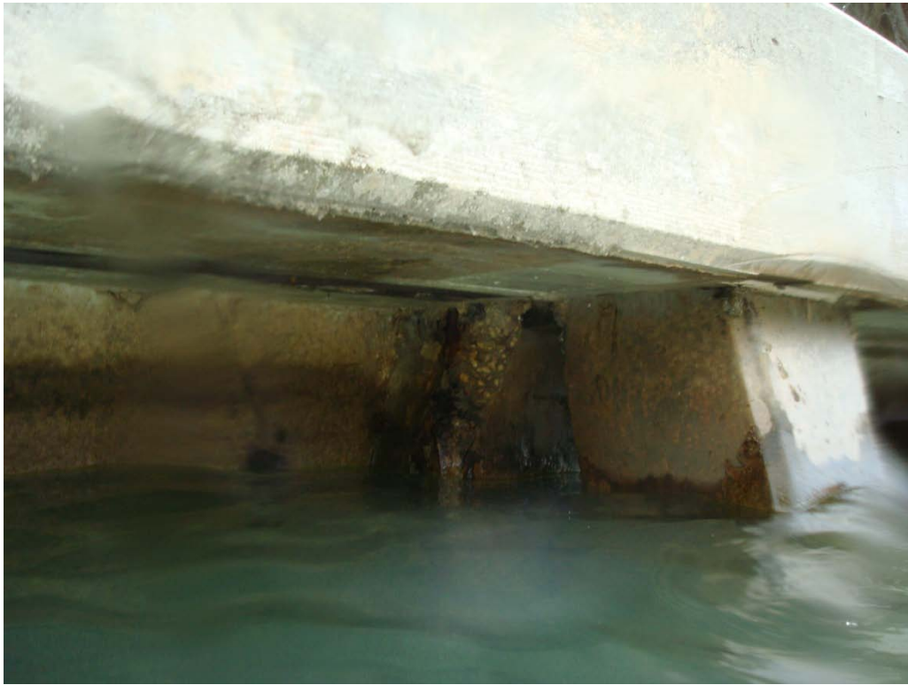
Photo 6.1: Exposed Steel Reinforcement
