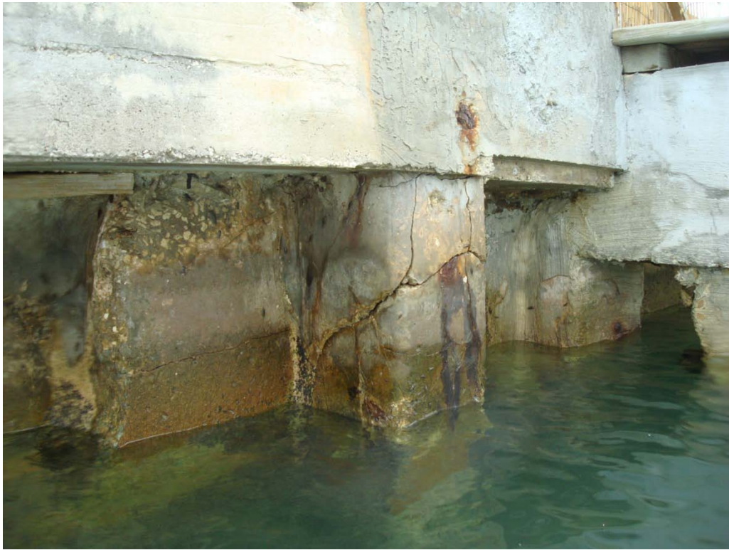
Photo 11.1: Cracking in King Pile
