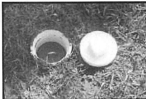
Figure 4.14 LDL Plug Installed in Cleanout (Courtesy, USSI, Inc)
