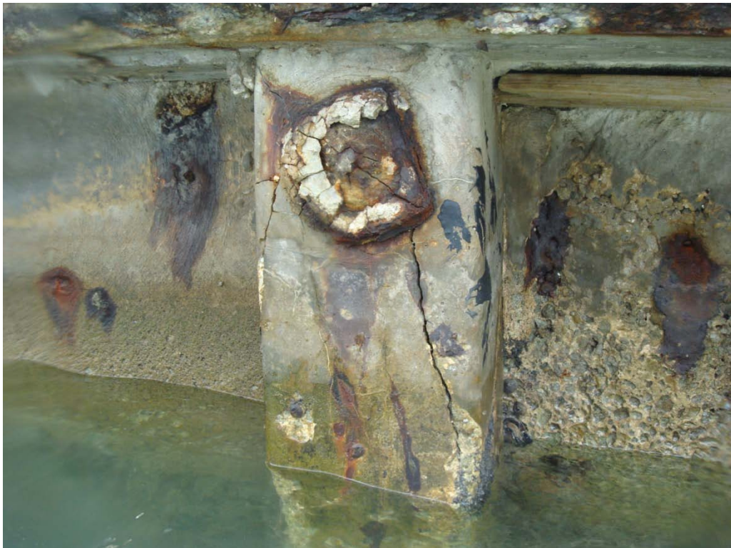
Photo 11.2: Cracking in King Pile, Spalling Cap
