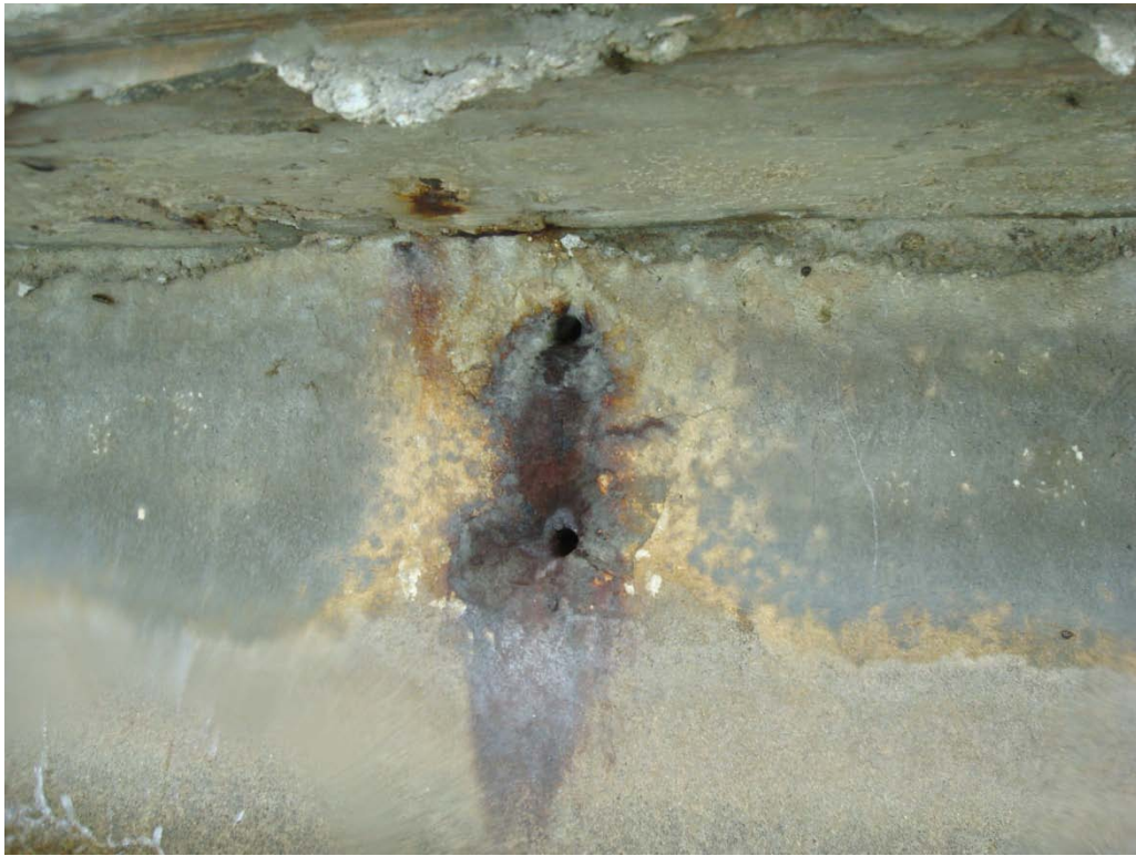
Photo 11.5: Rusted Steel Reinforcement Leaking Through Wall
