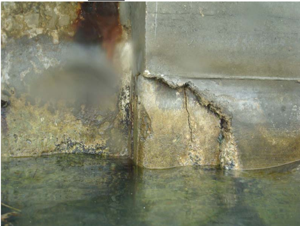
Photo 8.2: Cracks Observed in H-piles
