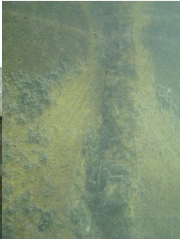
Photo 9.3: Vertical Shear Crack
