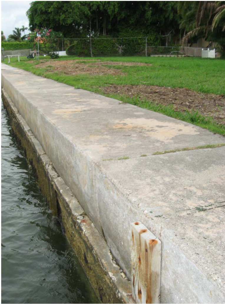
Photo 2.1: Concrete Bulkhead with Asbestos-Concrete Sheets
