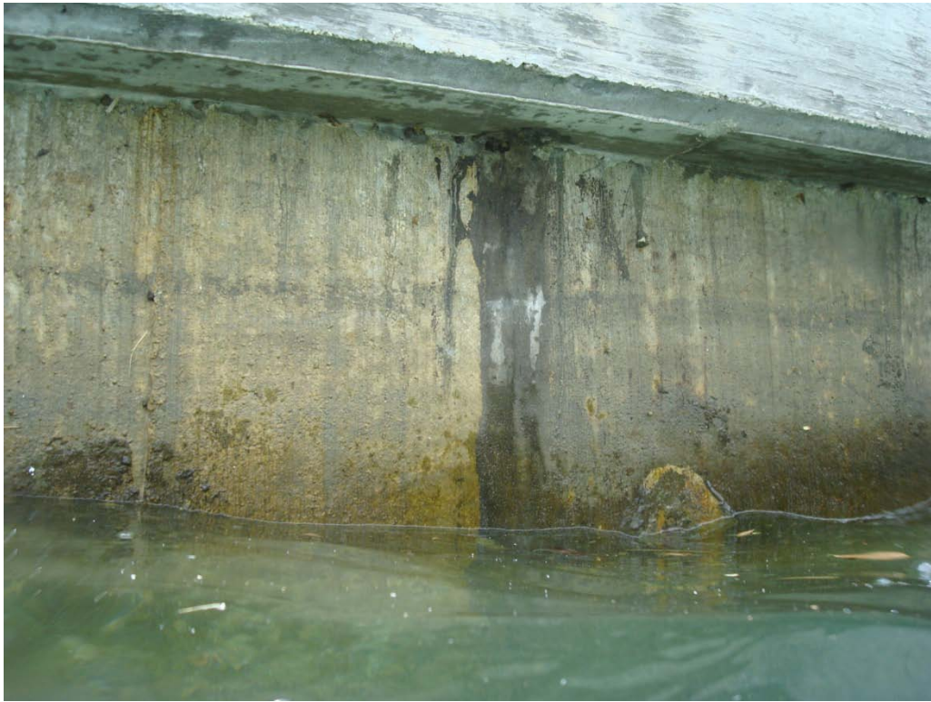
Photo 7.1: Joint between Concrete Sheet Piles
