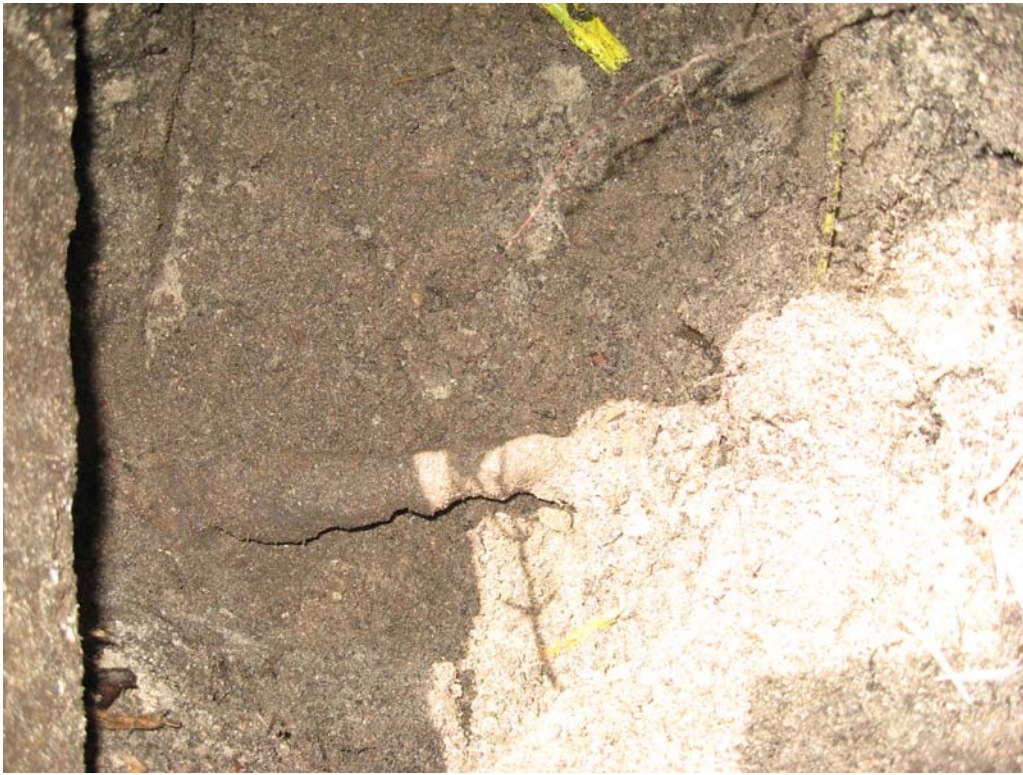
Photo 12.3: Excavated Tieback Rod in Good Condition
