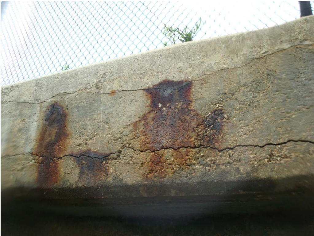
Photo 12.4: Longitudinal Spall Cracking in Cap, Rusted Reinforcement
