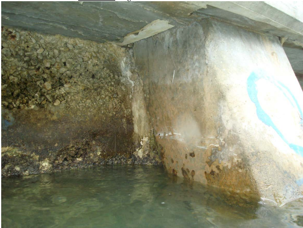
Photo 5.4: Degraded Concrete Sheet Piles
