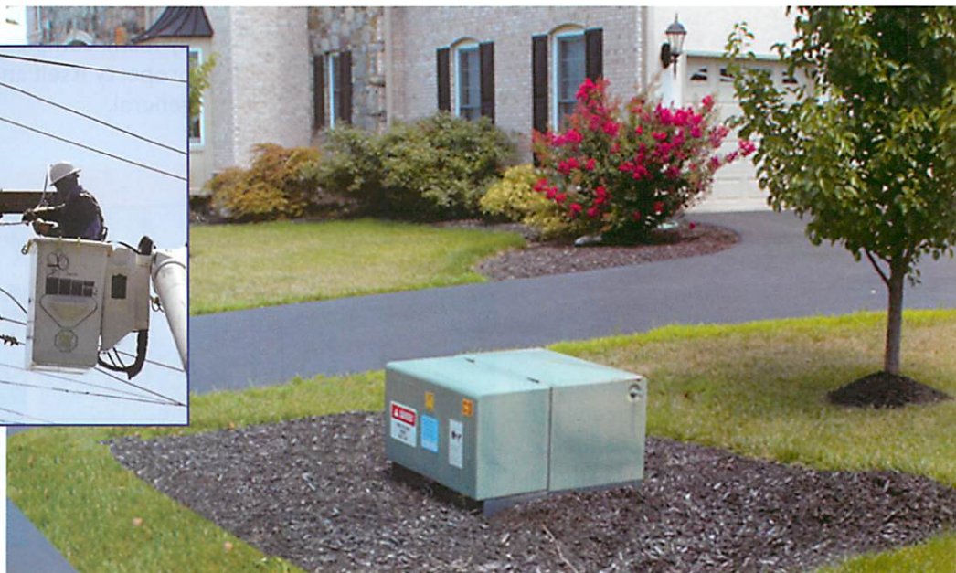
Overhead lines and poles (inset) would be replaced by access boxes located on property lines (shown at right).
