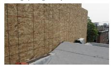
Figure 5. This interface between a rising wall and an existing roof will require careful detailing to exclude water. Any active chimney flues will also need to be extended above the new, higher roof line.
