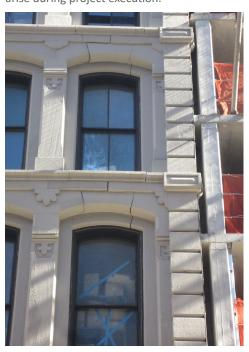
Figure 1. Cracking and displacement of existing stone arches due to foundation settlement associated with adjacent construction. New floor slabs also extend into a required seismic gap, where they can apply damaging earthquake loads to the existing building.
