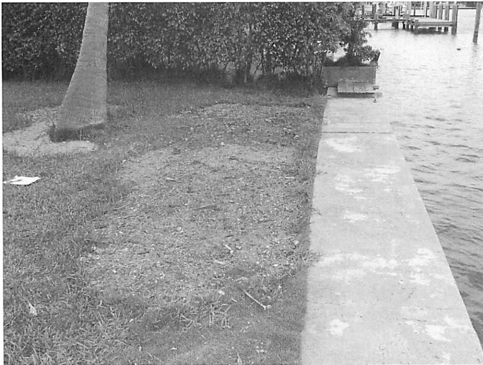
Photo 2.2: Recently Placed Imported Fill
