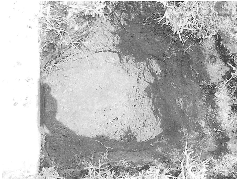
Photo 10.2: Concrete-Encased Tieback Rod
