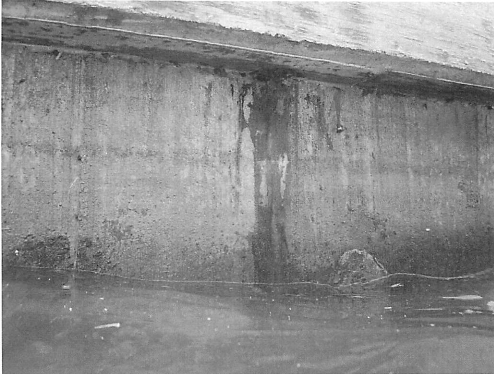
Photo 7.1: Joint between Concrete Sheet Piles
