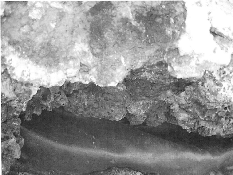
Photo 1.3: Geofabric Witnessed Through Wall
