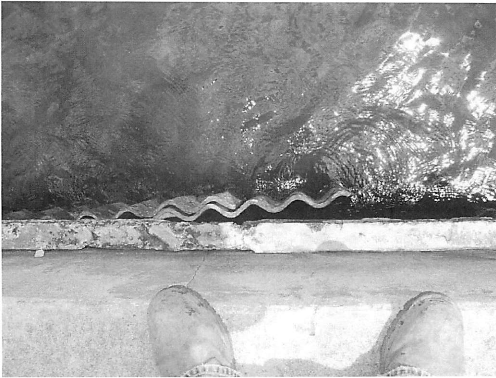
Photo 2.2: Asbestos-Concrete Sheet Piles In Front of Wall
