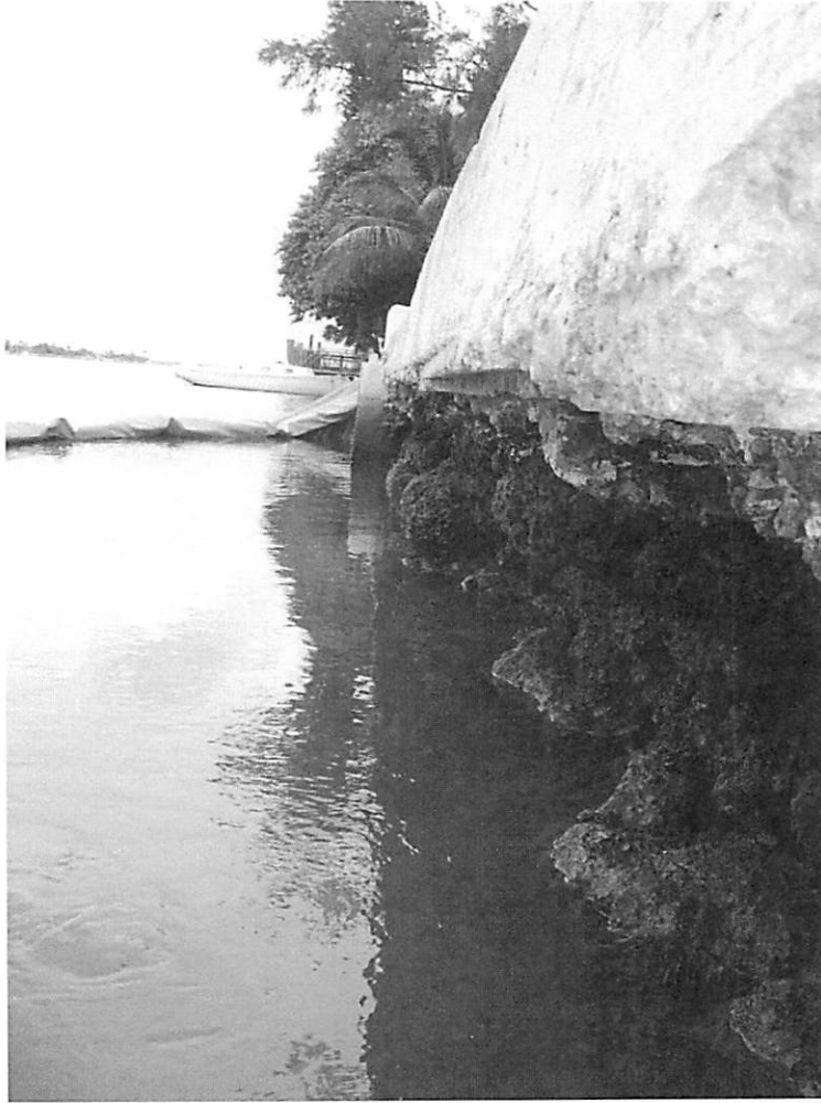
Photo 1.1: Native Stone Wall
