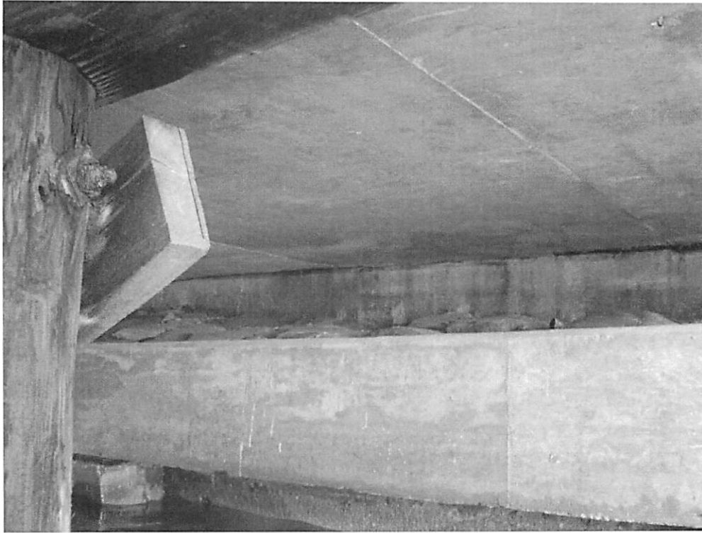
Photo 3.1: Concrete Cap In Front of Abutment with Backfill
