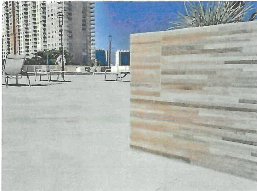
The amenities area received a new porcelain deck and wood-look mosaic planters.
