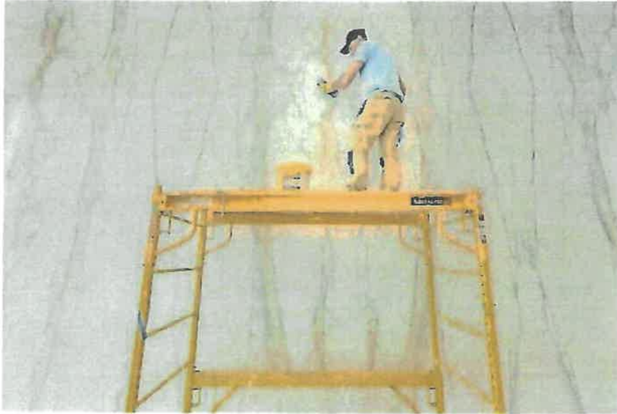
PH's Grigoris Iskritilis applies Sika Tile®-800 Unsanded Grout to huge Cafacatia slabs.
