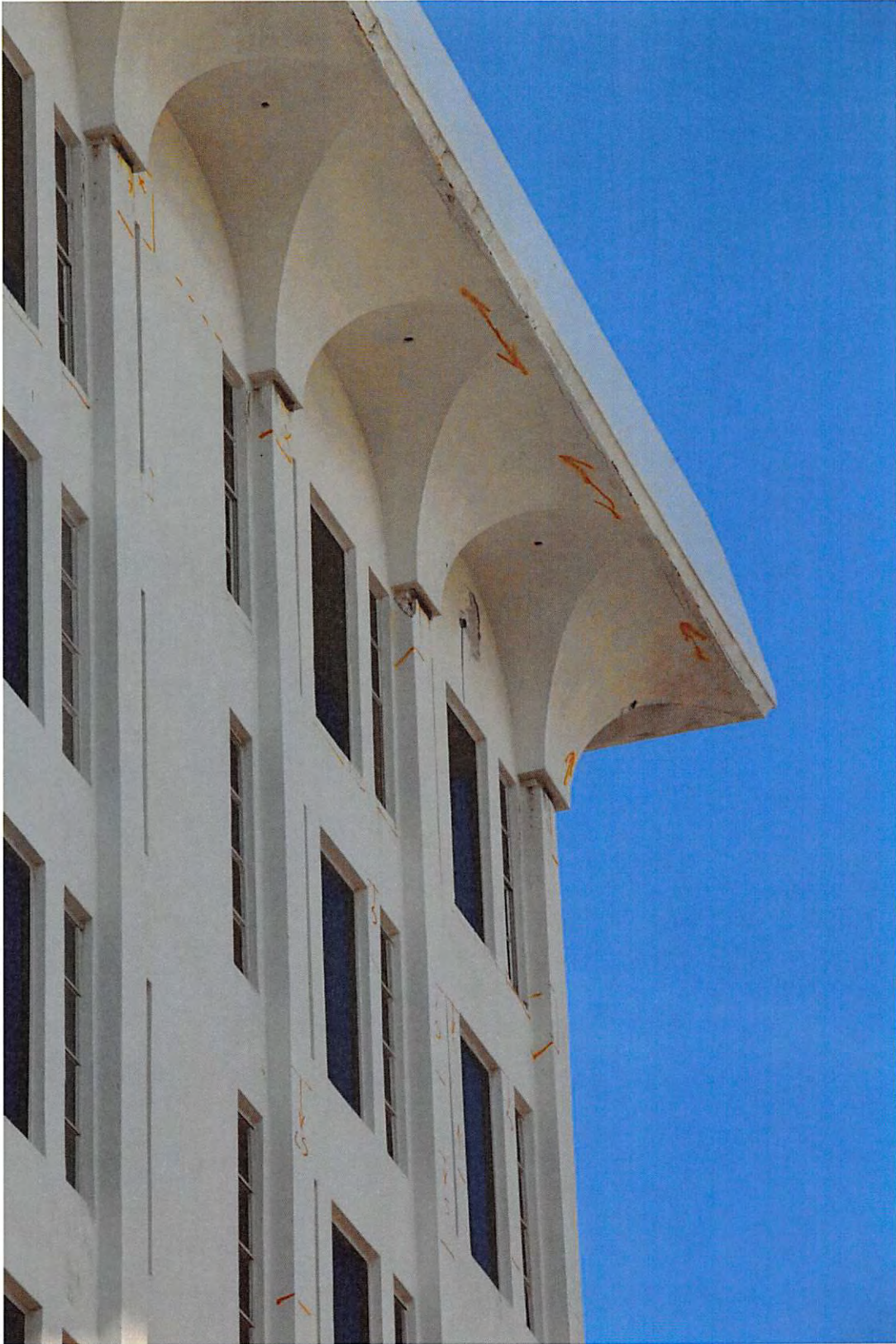
DETAIL VIEW OF WINDOW PATTERN AND PARAPET ARCHES.
