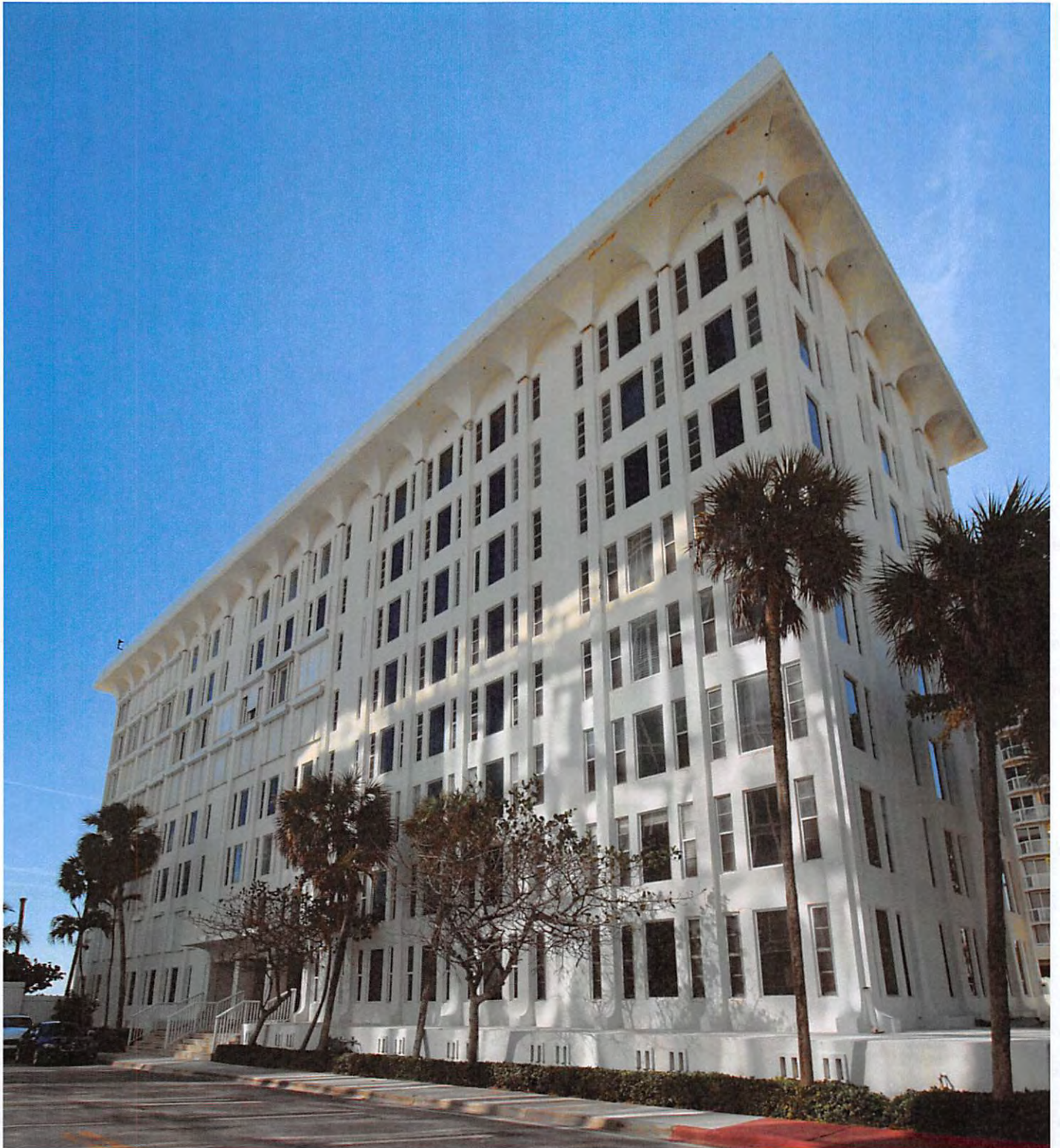
PANORAMIC VIEW OF NORTH (LEFT) ELEVATION AND WEST ELEVATION (RIGHT)
