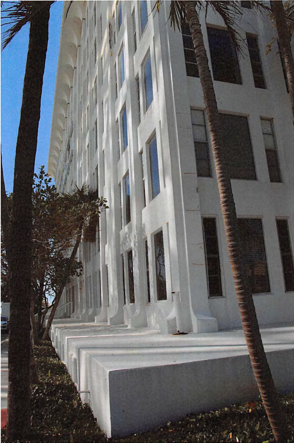
THE BUILDING SUPERSTRUCTURE COMES TO REST UPON A WIDE CONCRETE PLINTH THAT CONTAINS THE ENTIRE BUILDING.
