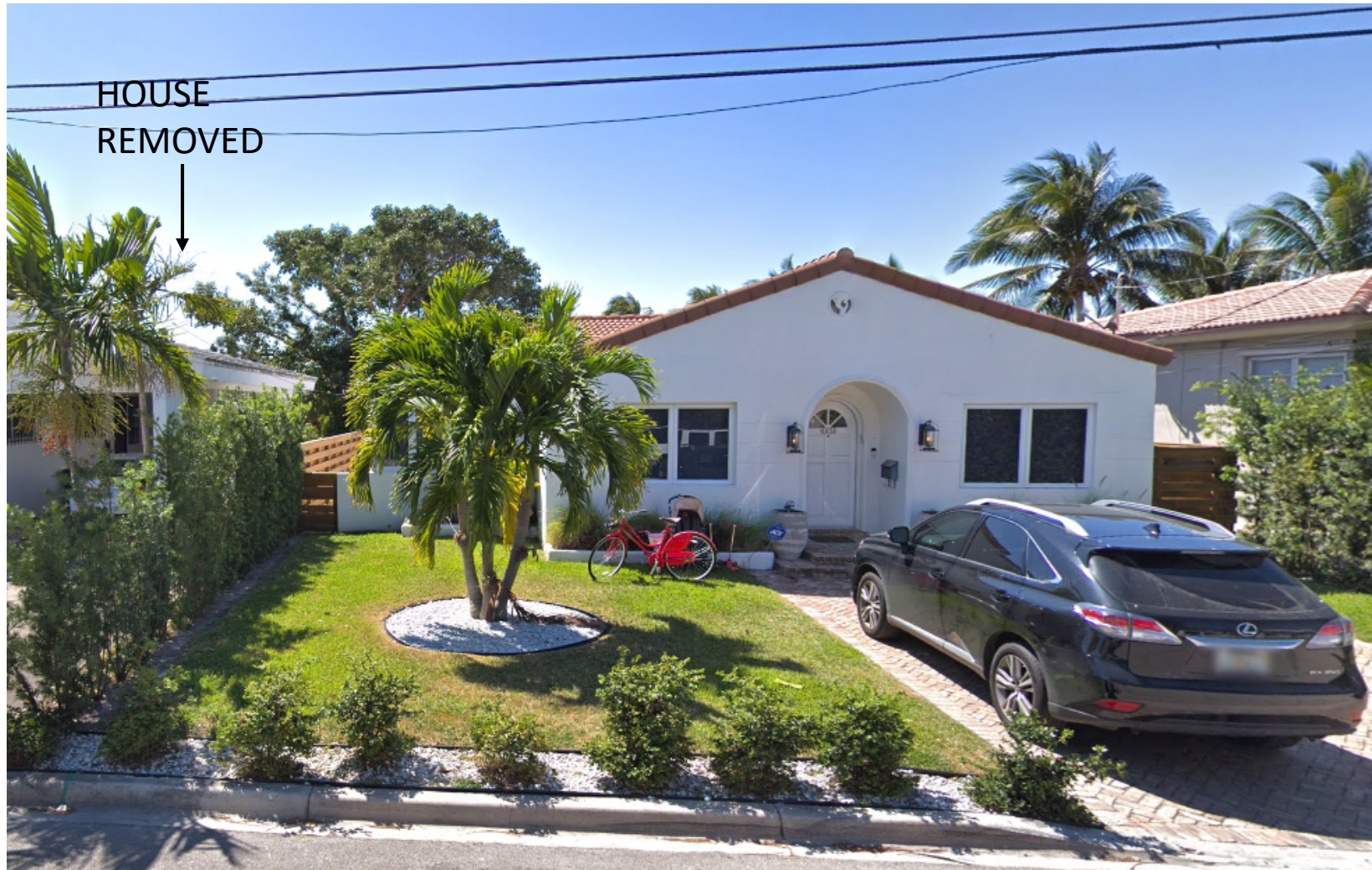
EXISTING PHOTO OF 8834 FROUDE AVENUE, SURFSIDE, FL 33154 THIS HOUSE IS ADJACENT TO THE NORTH SIDE
