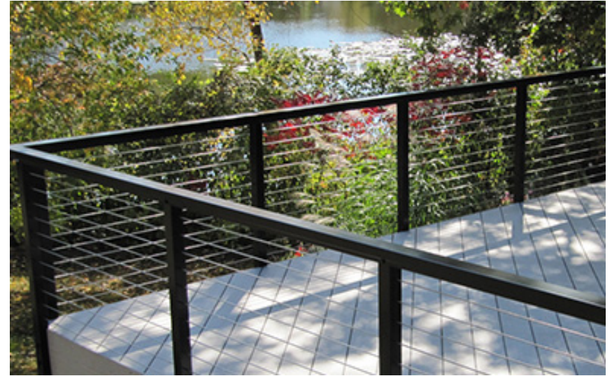
EXTERIOR BALCONY RAILINGS
