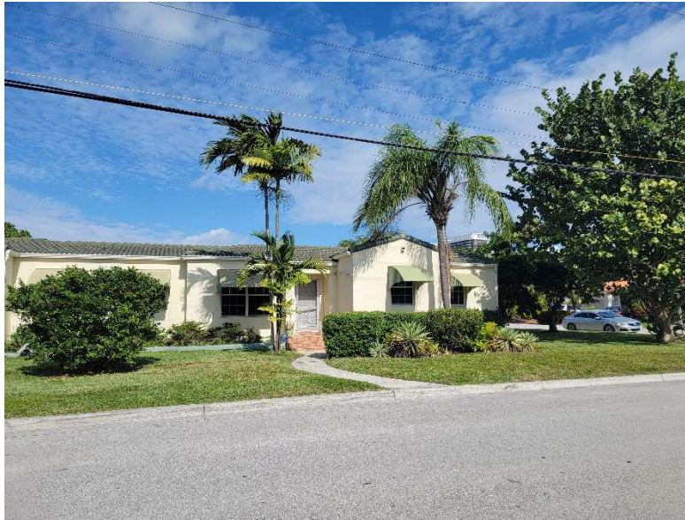
VIEW FROM 94 TH STREET
