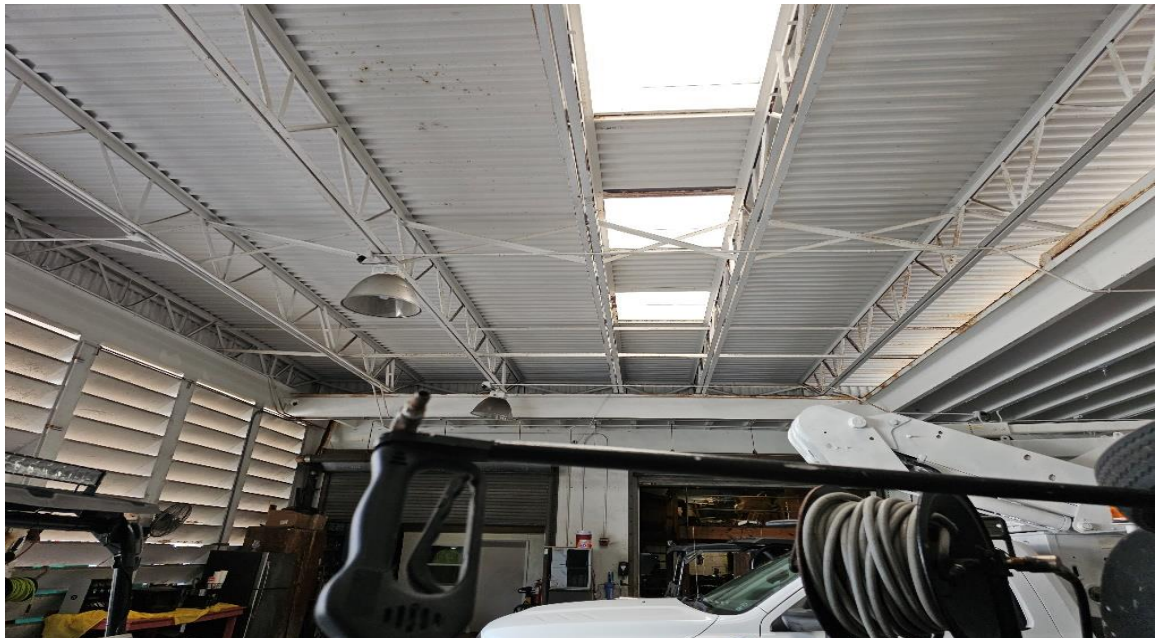
ROOF JOISTS AT INTERIOR YARD IN GOOD CONDITION
