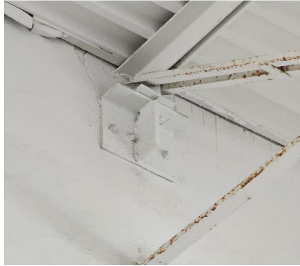
STEEL JOISTS CONNECTION IN GOOD CONDITION
