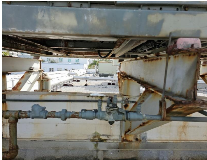
RUST OBSERVED ON THE CHILLERS SUPPORT PLATFORM BEAMS
