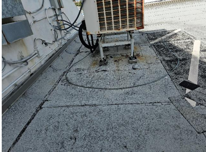
RUST OBSERVED AT RTU BASE CONNECTION
