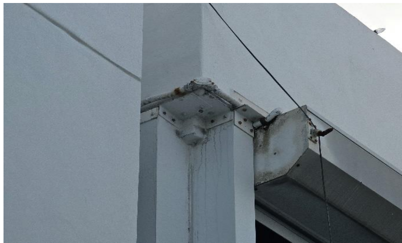
RUST OBSERVED ON EAST ENTRANCE STOREFRONT FRAMING
