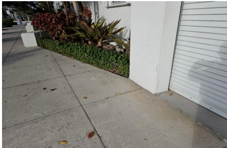
CRACKS OBSERVED AT DOOR JAMB
