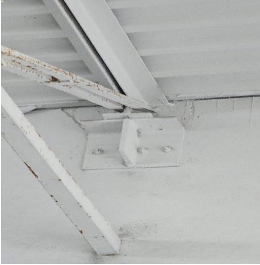
STEEL JOISTS CONNECTION IN GOOD CONDITION
