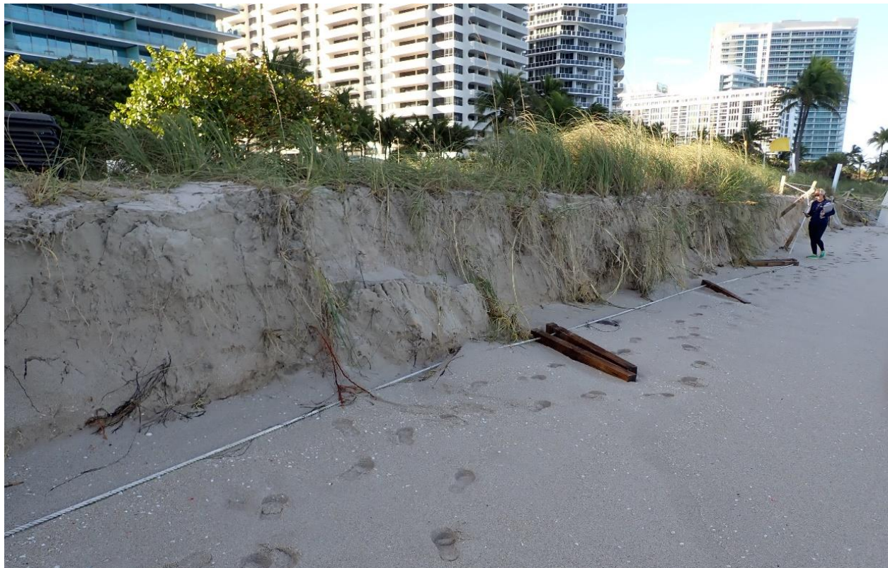
PHOTO 13. DISLODGED FENCE POSTS AND DUNE GRASSES (ACCESS 14-15)
