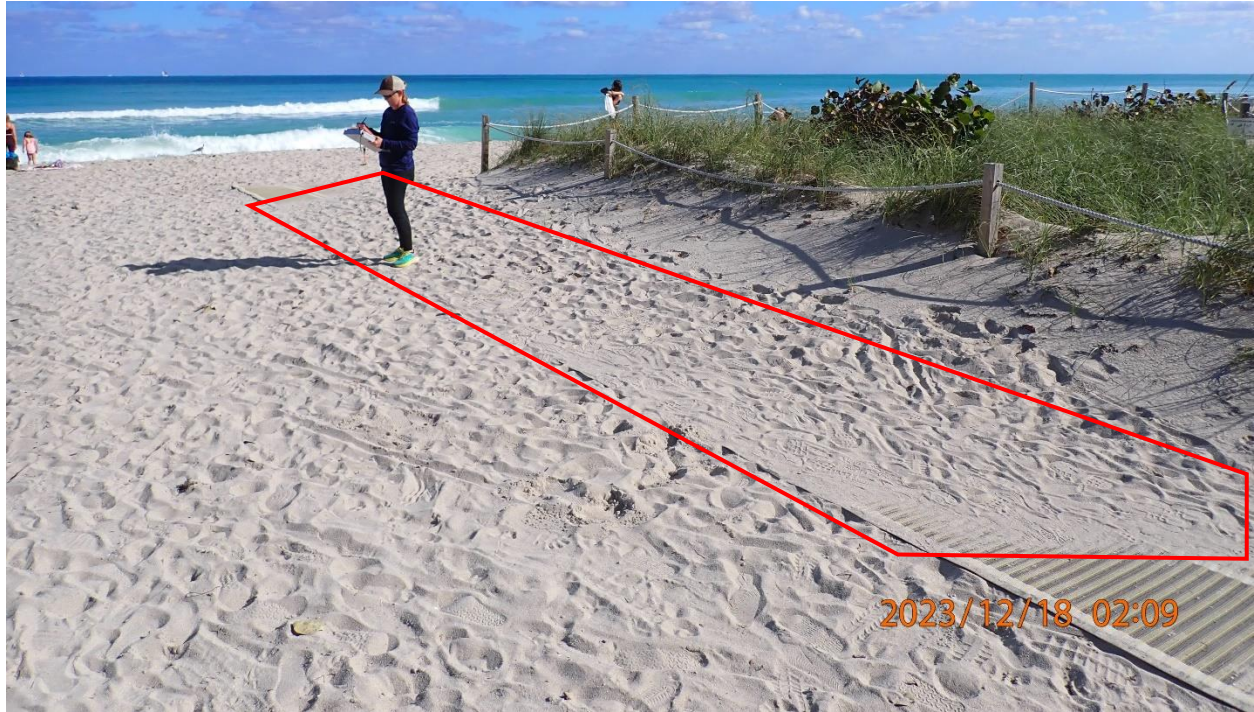
PHOTO 2. BURIED BEACH ACCESS MAT (ACCESS 1)
