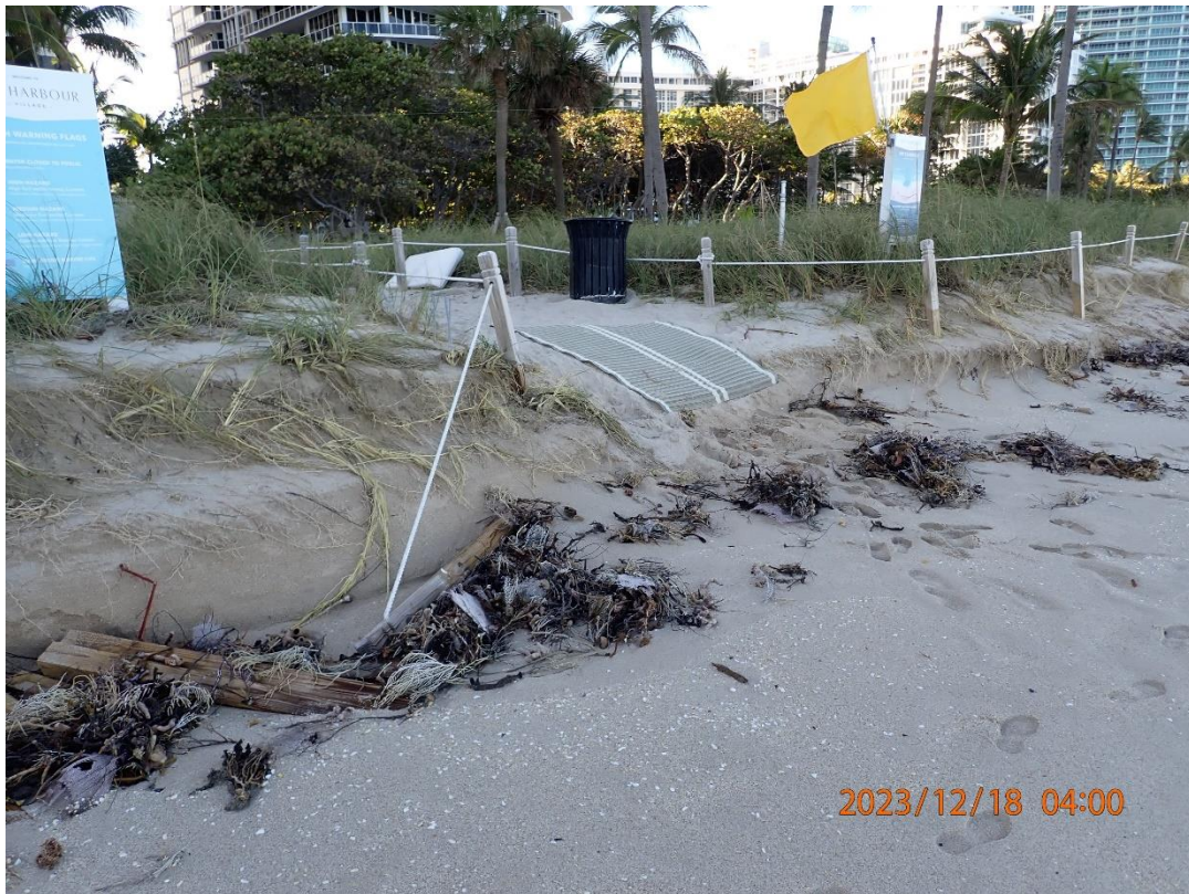
PHOTO 17. BEACH EROSION AT ACCESS 16
