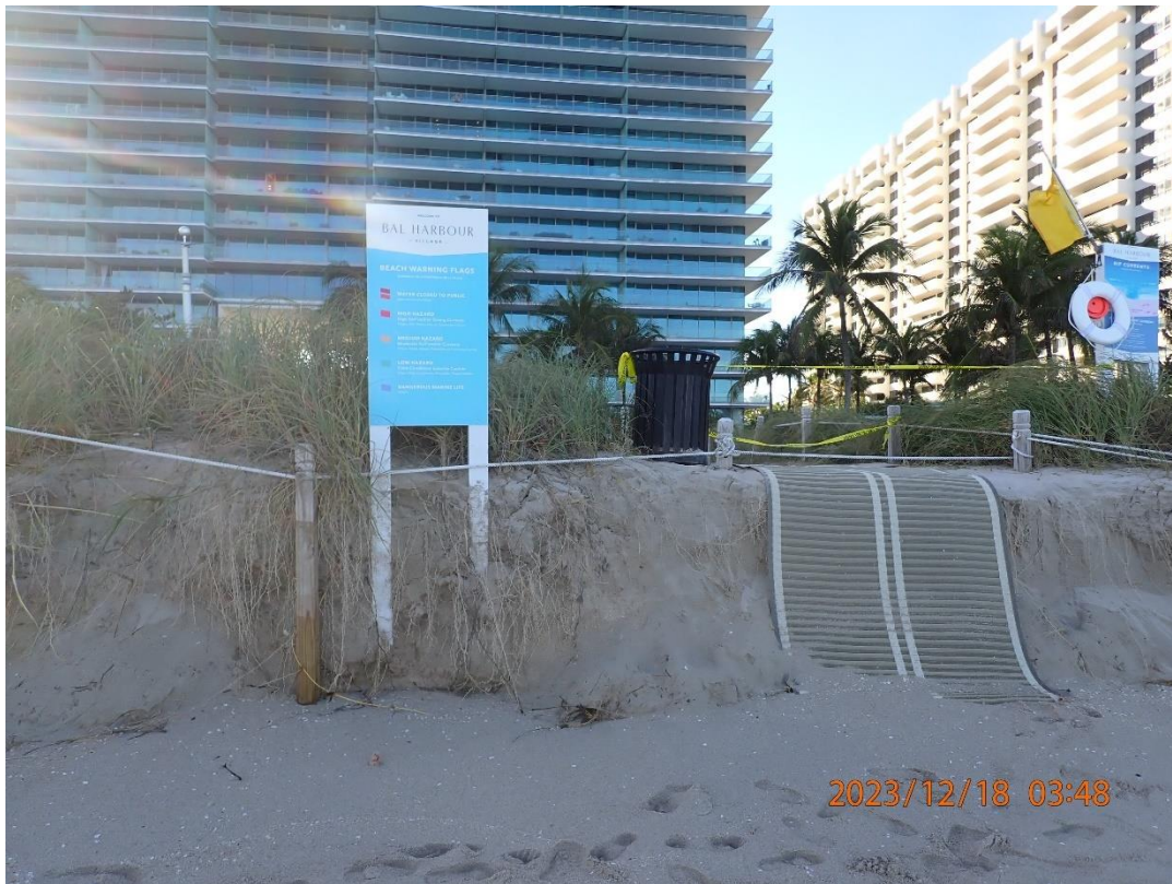
PHOTO 15. EXPOSED POSTS AND UNSAFE BEACH ENTRY (ACCESS 15)
