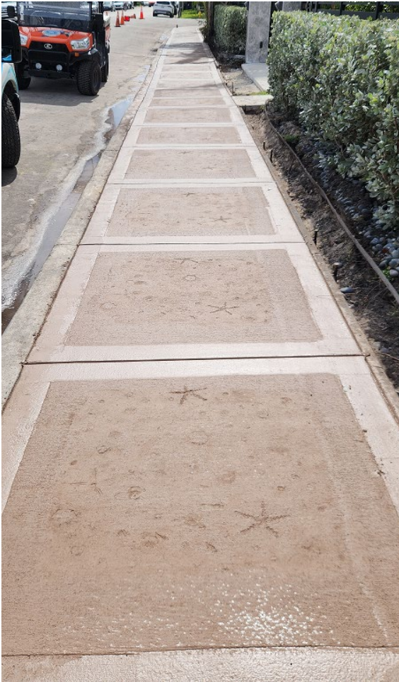
Finalized the 96 th Street sidewalk extension project
