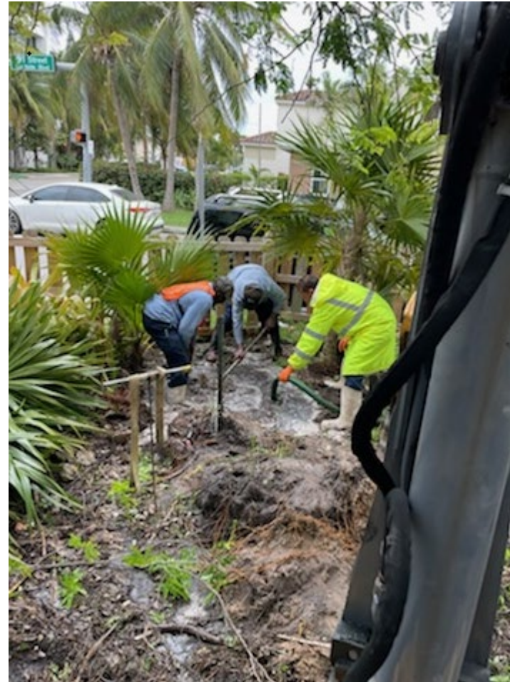
Utilities repaired a water break on 91 st Street & Harding Avenue
