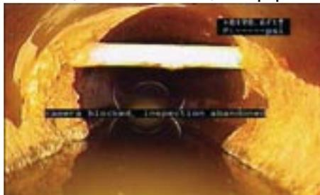
*Inspection camera shows a pipe section that is blocked and damaged.*
