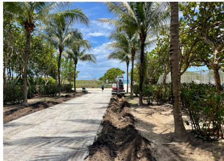
The department also started rebuilding the 90th Street Beach End walk path and nature area. Construction began on June 1st and will be completed this summer. The work consists of replacing the original damaged pavers, adding irrigation, adding turtle friendly lighting and improving the overall experience for town residents and visitors.
