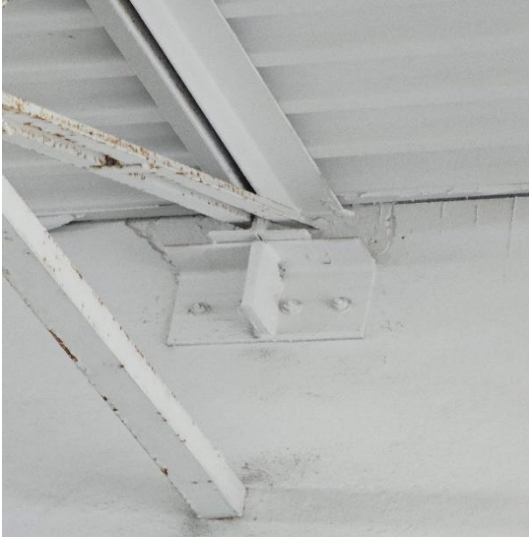
STEEL JOISTS CONNECTION IN GOOD CONDITION
