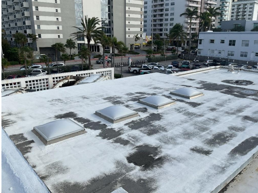
EAST LOWER ROOFING SYSTEM SHOWS BUBBLING AND SIGNS OF DETERIORATION
