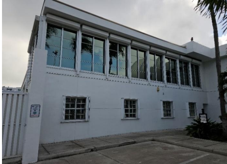
BUILDING EAST FAÇADE IN FAIR CONDITION
