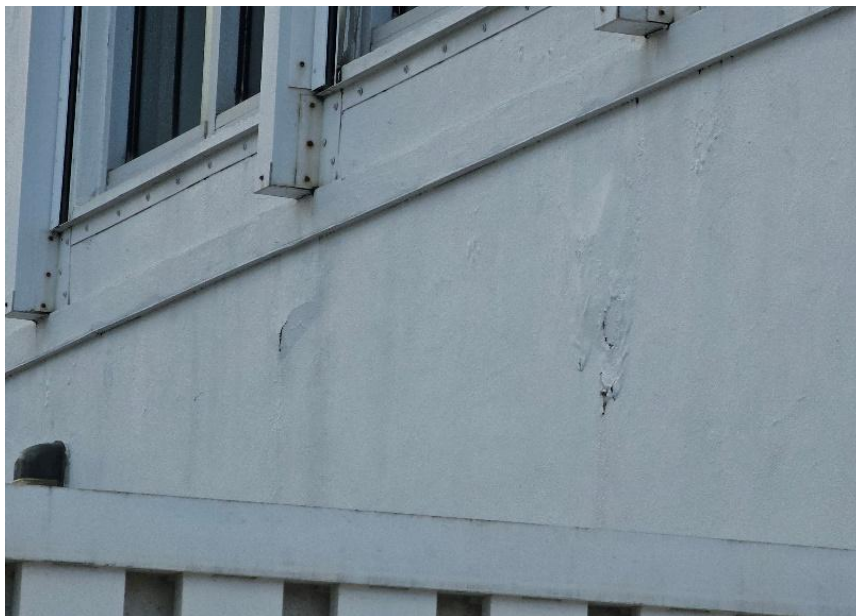
EAST FAÇADE SHOWS SIGN OF STUCCO PEELING AND DETERIORATION
