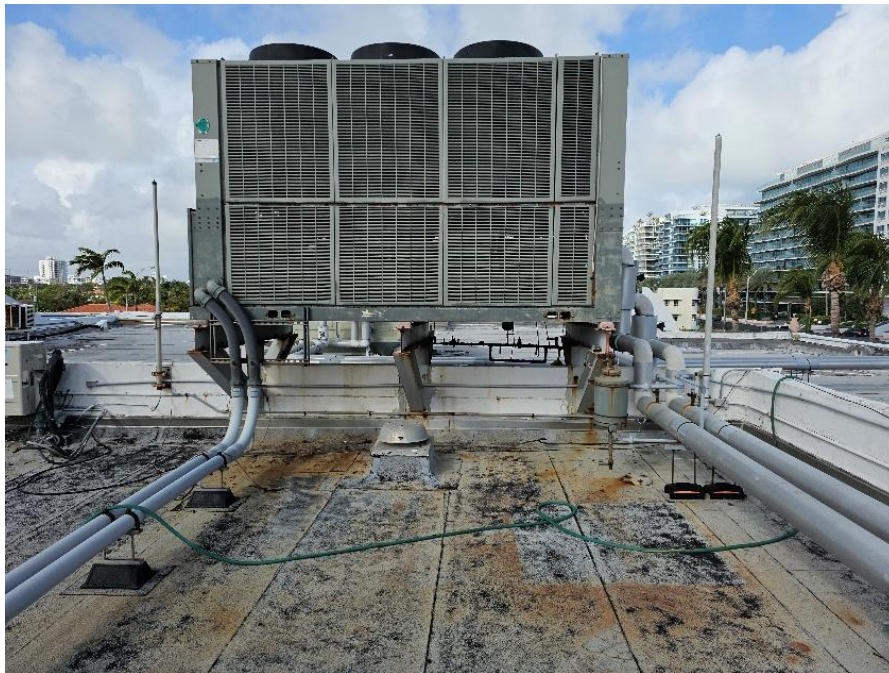
LOSS OF MEMBRANE AND CRACKING WAS OBSERVED IN THE ROOFING SYSTEM
