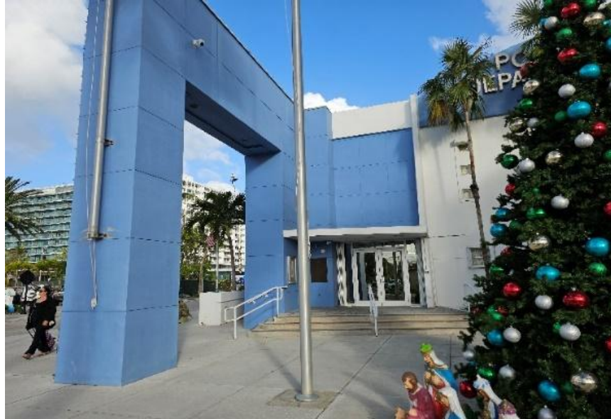
BUILDING WEST ENTRANCE WALL IN GOOD CONDITION
