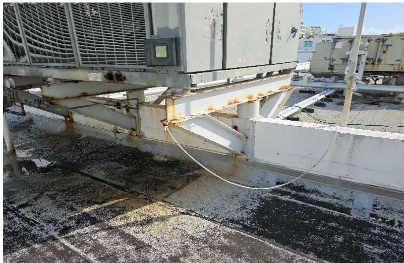
RUST WAS OBSERVED ON THE CHILLERS SUPPORT PLATFORM
