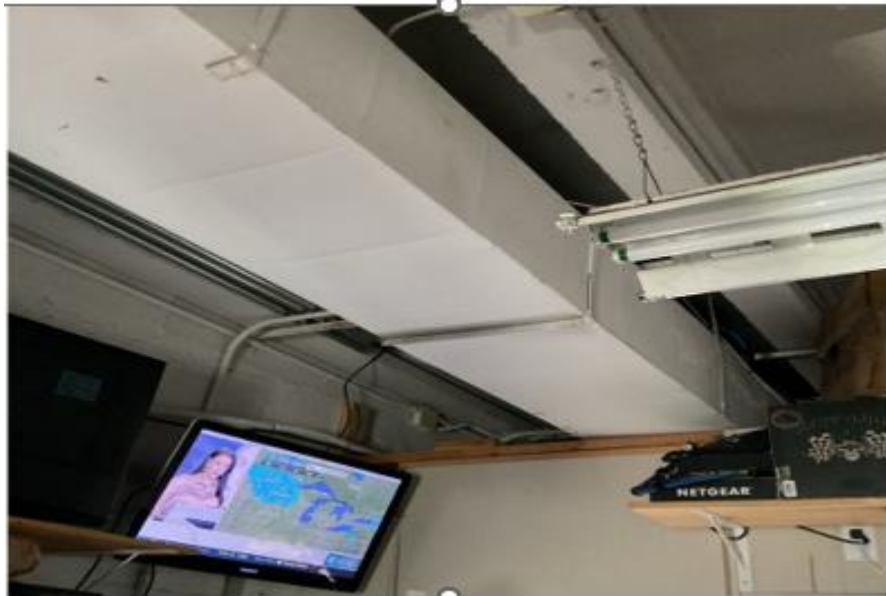
TYPICAL ELEVATED CONCRETE BEAM IN GOOD CONDITION
