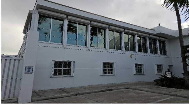
EAST FAÇADE WINDOWS IN GOOD CONDITION
