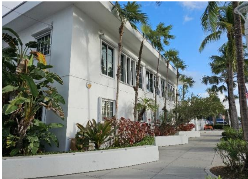
BUILDING WEST FAÇADE IN GOOD CONDITION
