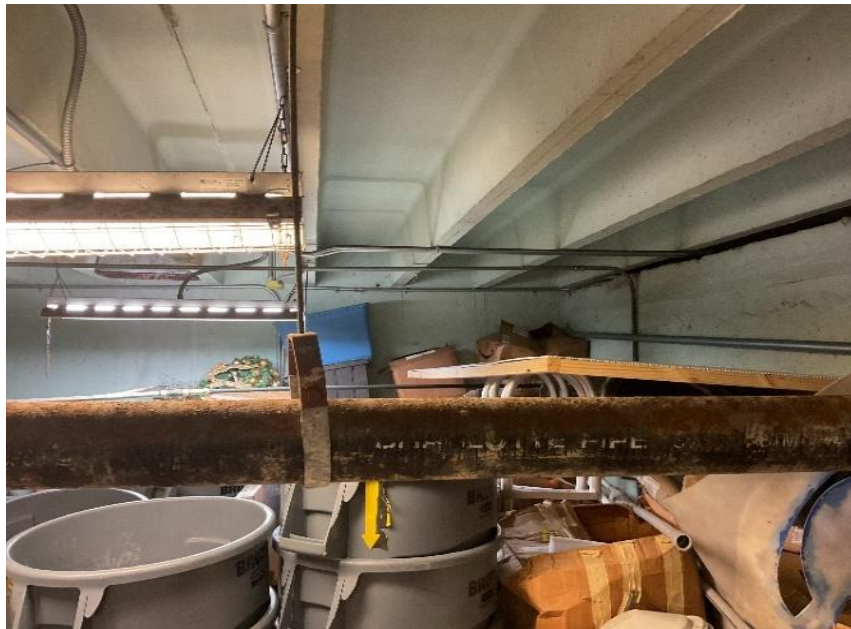
FLOOR DOUBLE TEES IN GOOD CONDITION
