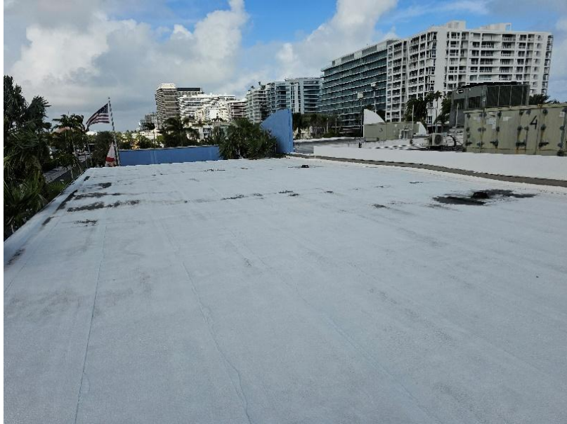
WEST ROOFING SYSTEM IN FAIR CONDITION
