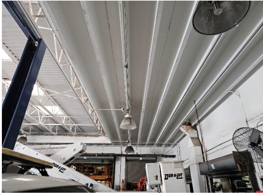
ROOF DOUBLE TEES AT INTERIOR YARD IN GOOD CONDITION
