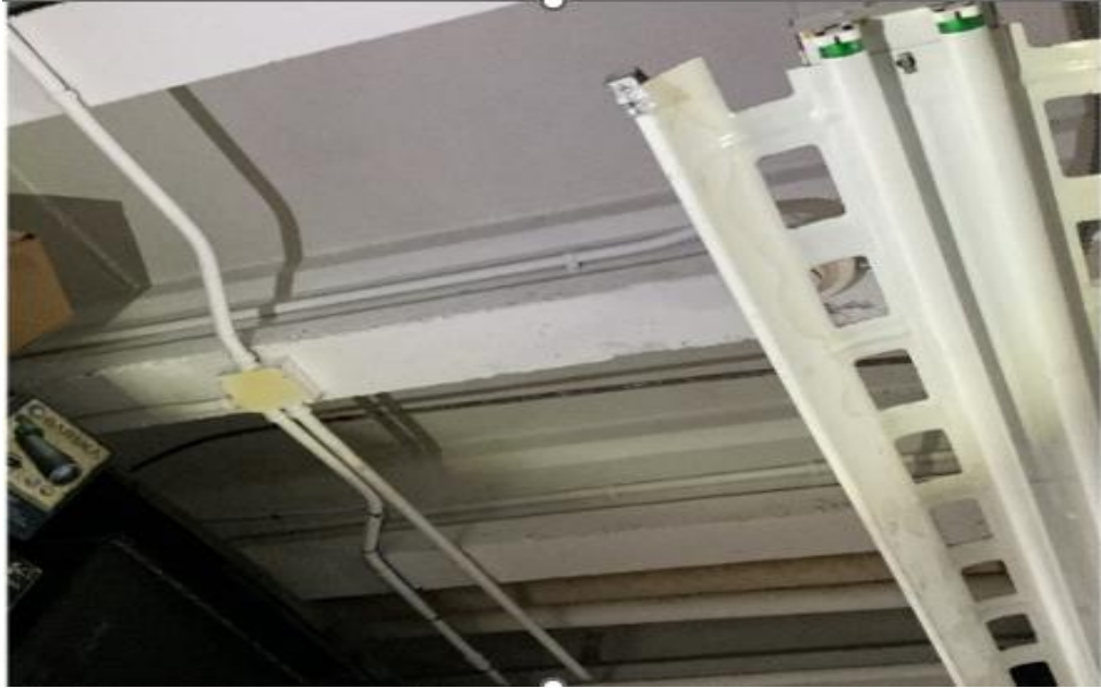
INTERIOR FLOOR PRECAST JOISTS IN GOOD CONDITION
