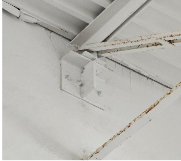
STEEL JOISTS CONNECTION IN GOOD CONDITION
