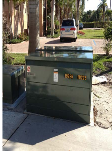
Picture 5 – Vista switch cabinet
