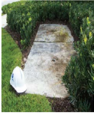
Picture 4 – Underground feeder splice box
