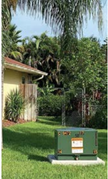
Picture 1 – Single phase transformer box
